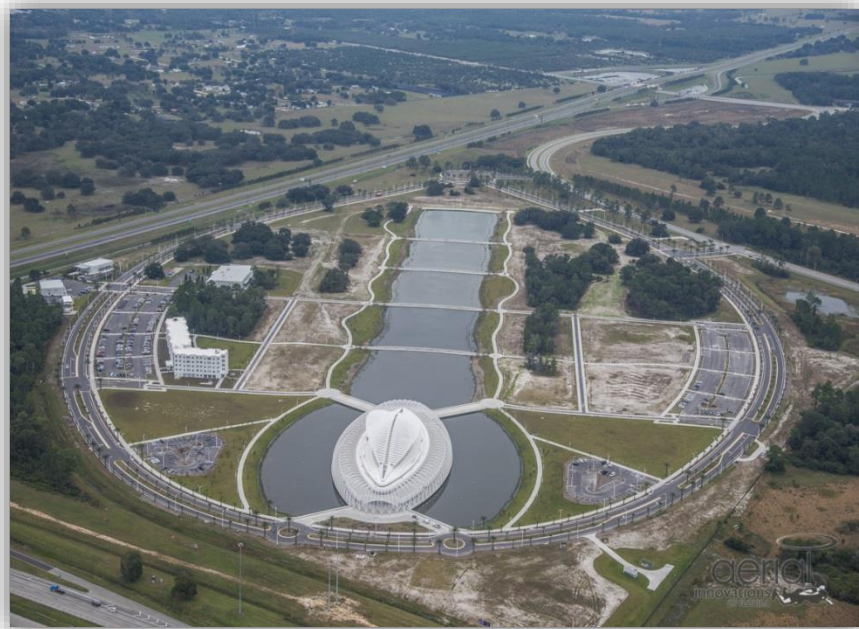
Florida Polytechnic University Campus View
