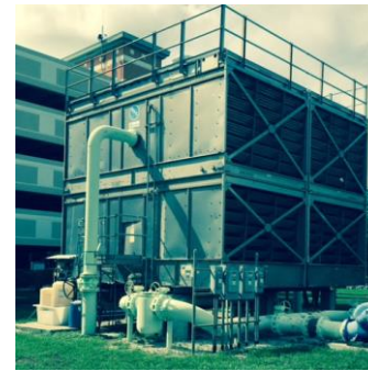
Cooling Towers 5 Constructed in 2007
