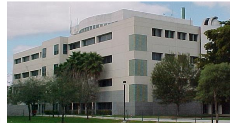
Science – bldg. 43 128,000 GSF
