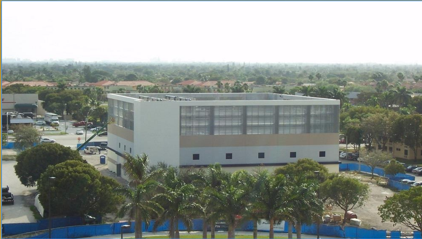
Satellite Chiller Plant Facility Partially Completed February 2013
