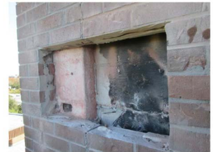
tower waterproofing – deteriorating and not consistently applied, no vapor barrier, no insulation
