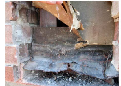
deteriorating substrate, flashing, no insulation, no vapor barrier
