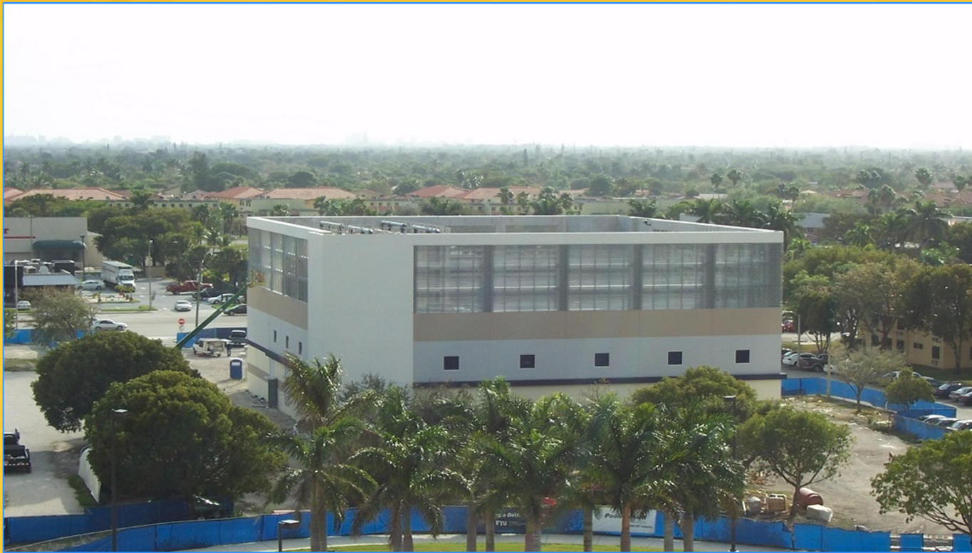
Satellite Chiller Plant Facility Partially Completed February 2013
