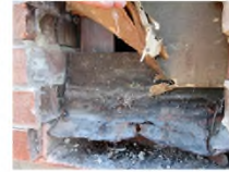
deteriorating substrate, flashing, no insulation, no vapor barrier
