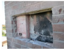
tower waterproofing – deteriorating and not consistently applied, no vapor barrier, no insulation
