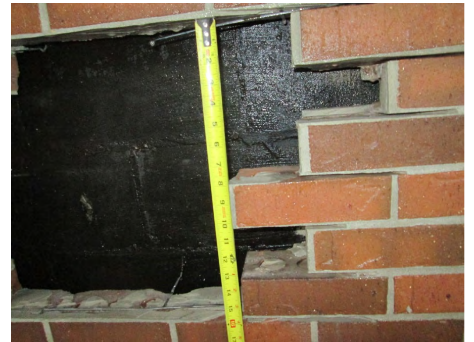
Vertical tie spacing measured at approximately 15-inches on center
