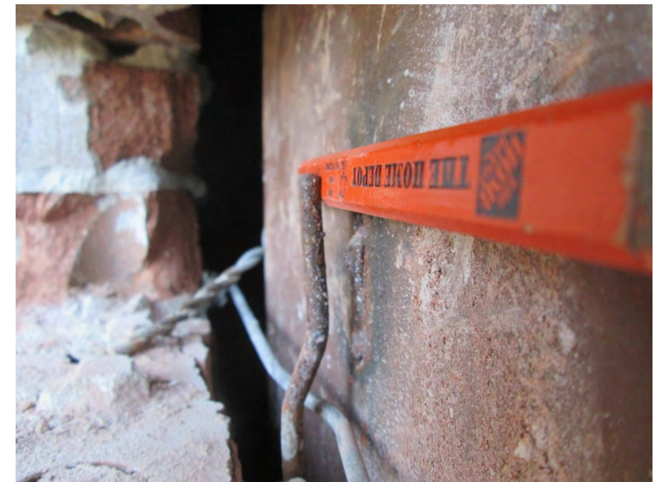
View of broken weld at wire loop connection to steel tube column
