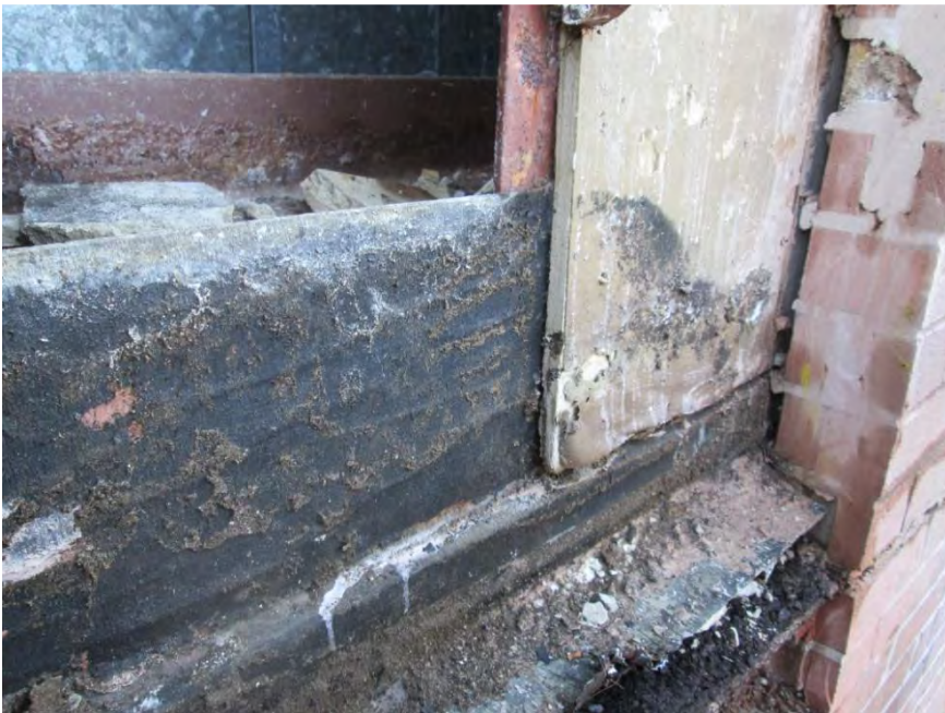
S46 - Cavity wall waterproofing consisting of gypsum sheathing and discontinuous flashing
