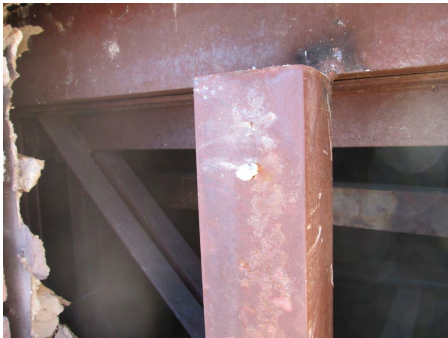
Uninstalled corrugated metal tie for lateral support of brick cladding
