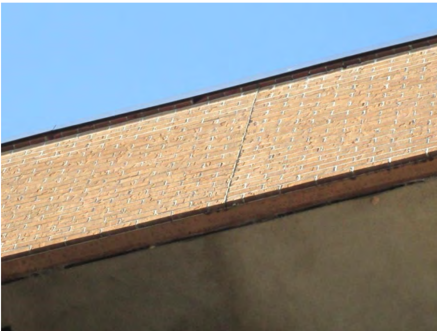
S42 - Extruded sealant failure in parapet wall expansion joint
