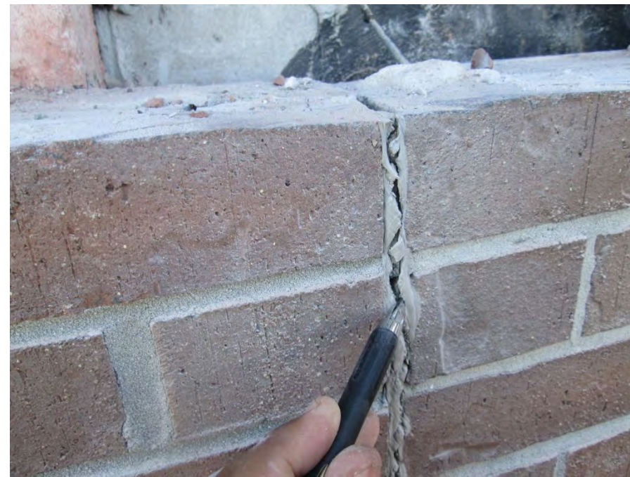
Failed joint sealant at expansion joint
