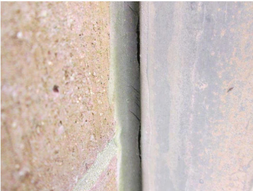
S44 - Sealant failure at brick façade transition to louver framing
