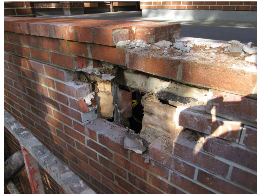
Deflected brick and separated mortar (through wall fabric flashing acts as bond breaker in masonry bed joint)
