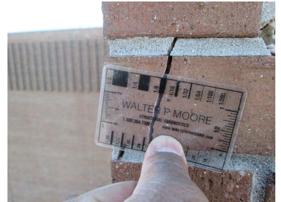
Brick crack width measured as 1/8- inch
