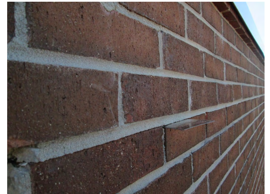
Mortar separation due to through-wall fabric acting as bond breaker
