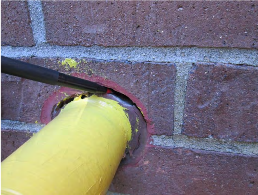
S43 - Failed sealant at through-wall pipe penetration
