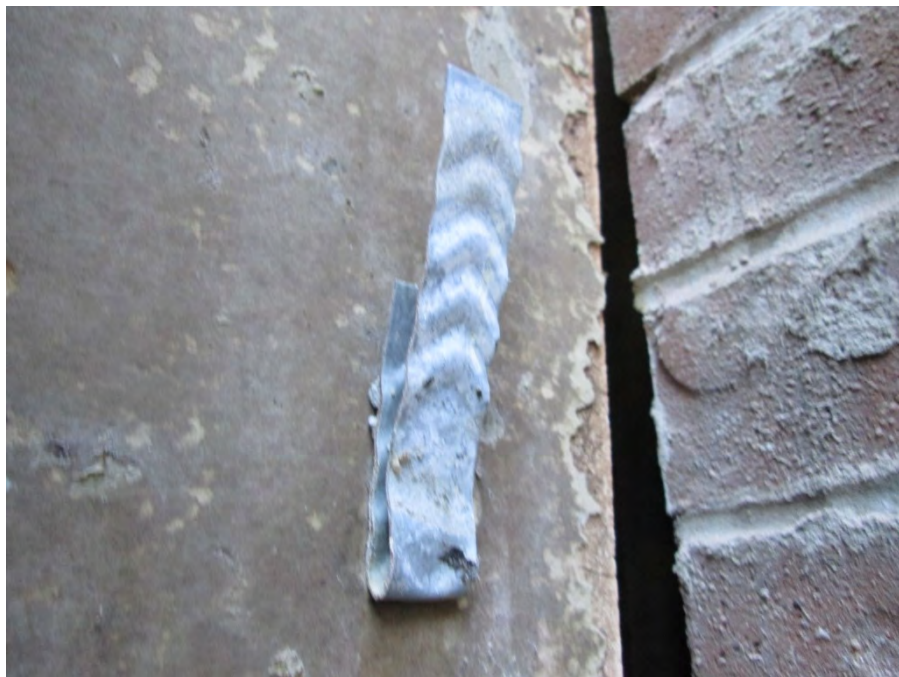
Corrugated metal tie not installed in brick masonry bed joint during original construction
