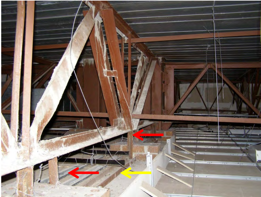
S83 - General view looking along top of wall shown in previous photo (red arrows highlight vertical angles hung from bottom chord of joist and welded to steel channel (yellow arrow) at top of window below)
