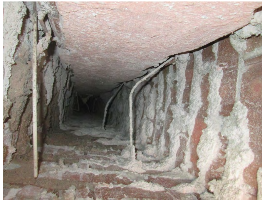
Wire ties for lateral attachment of brick cladding
