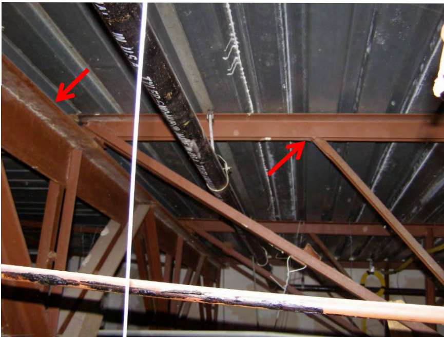
S58 - General view of floor joist (right arrow) bearing on top chord of joist girder (left arrow)
