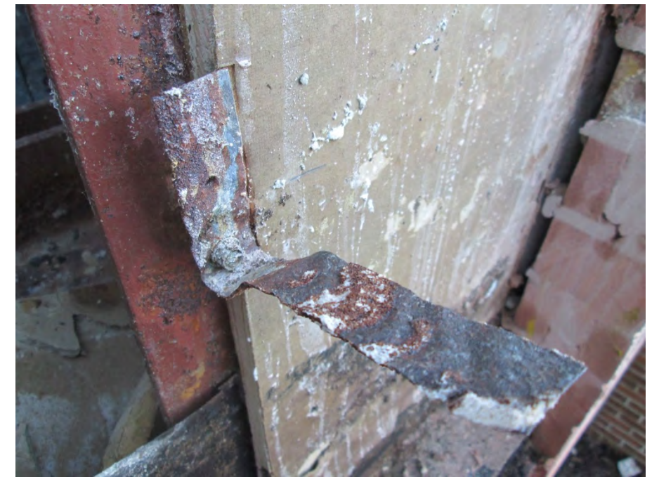
Corroded corrugated metal tie
