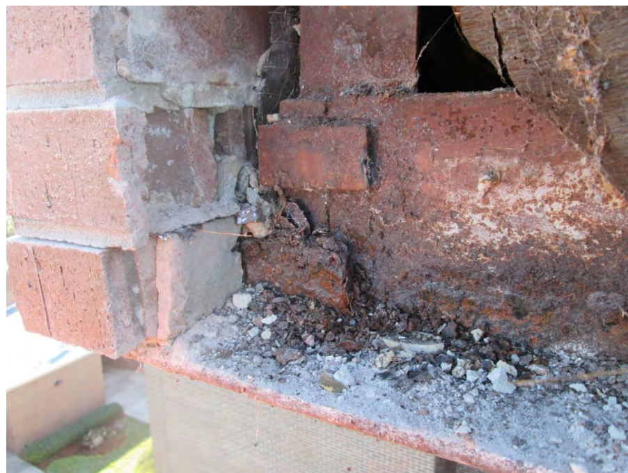
Corrosion distress of discontinuous shelf angle (note splice in shelf angle at location of rotated brick)
