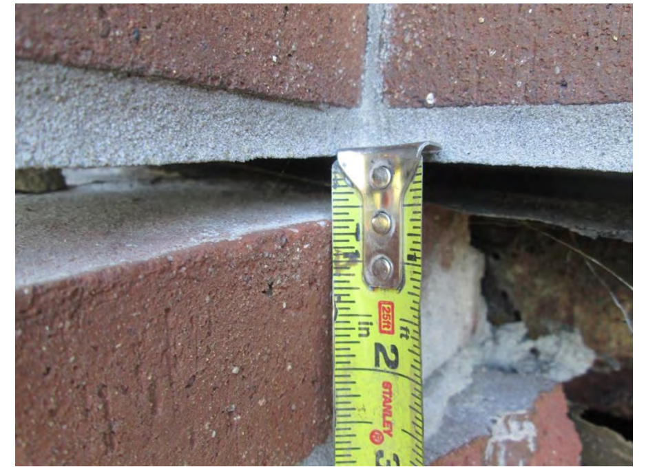
Separated mortar gap measured as approximately 5/8-inch
