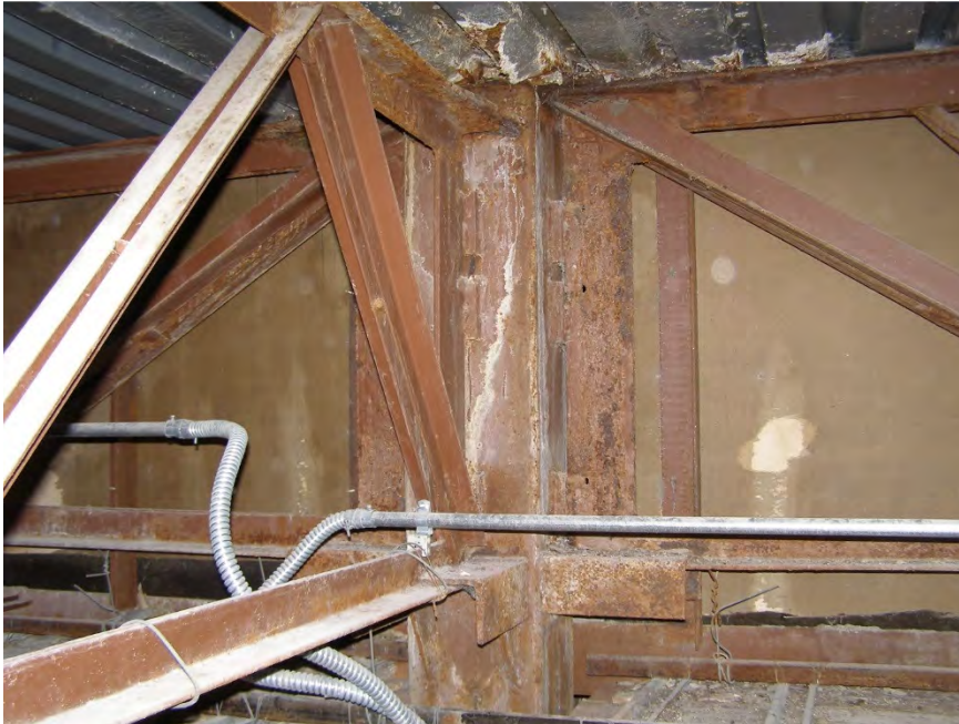
S67 - General view of corrosion of deck and steel framing below Level 2 exterior corridor
