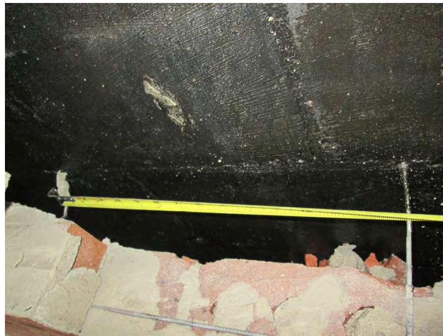
Vertical tie spacing measured at approximately 15-inches on center
