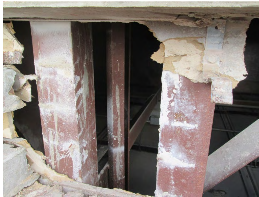
Surface corrosion noted at corrugated metal tie
