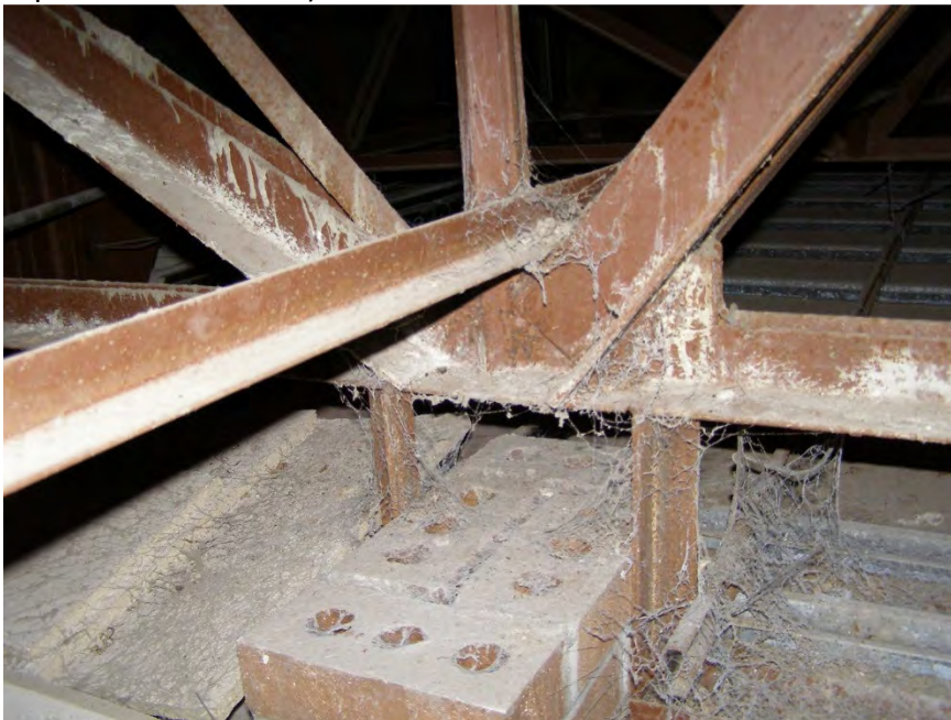
S84 - Top of discontinuous ungrouted, unreinforced brick pilaster at location shown in previous photo
