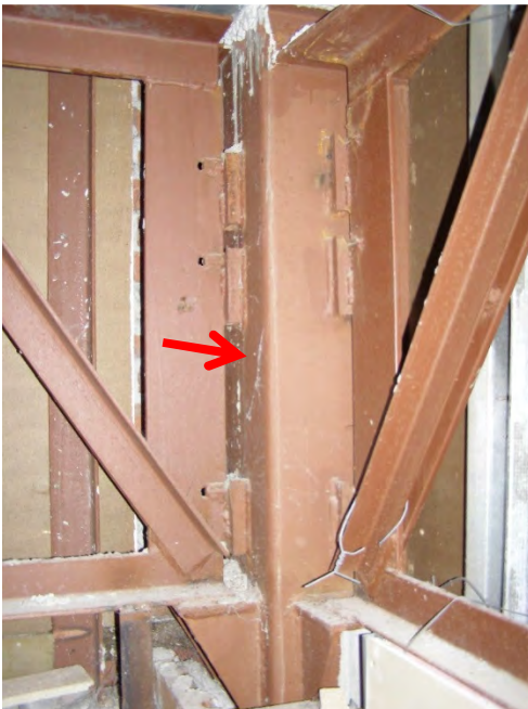
S56 - Arrow highlights typical 10"x10" tube steel column
