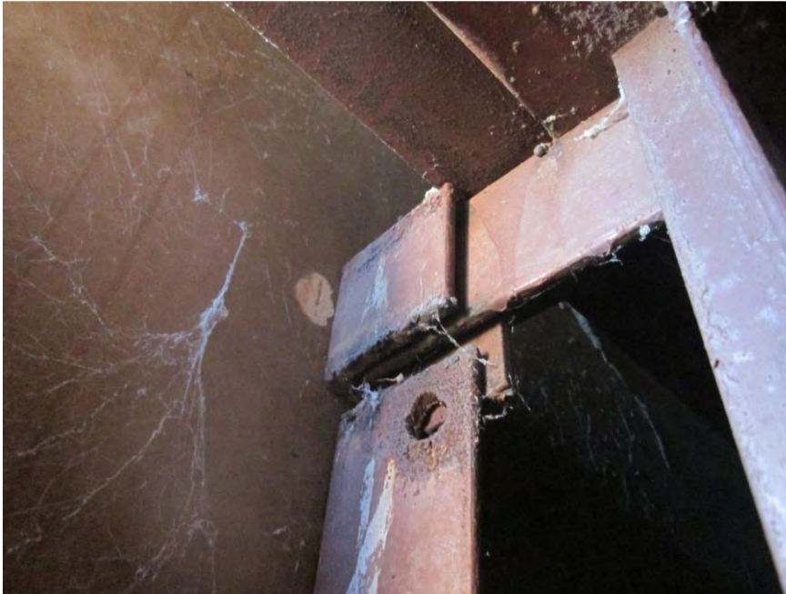
S25 - Backup vertical steel angles welded using steel tab plates to built-up joist bracing framing
