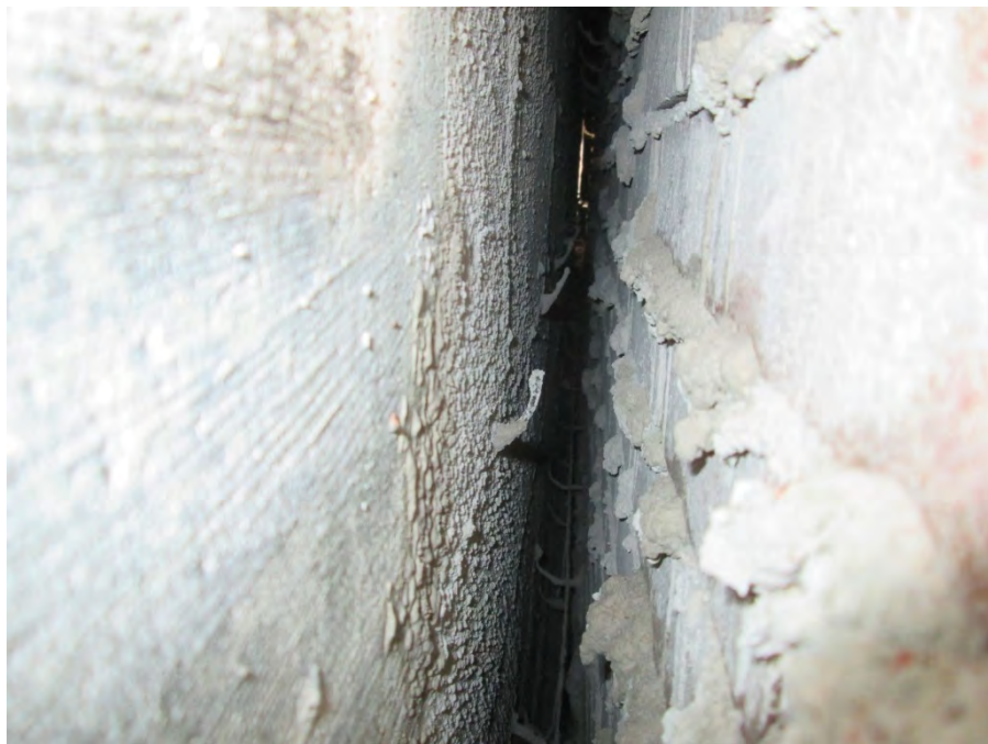
Cut ties of ladder reinforcement projecting from CMU wall backup
