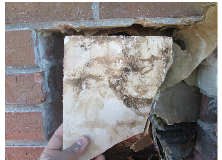
Signs of previous water infiltration as evidenced by water staining of gypsum sheathing
