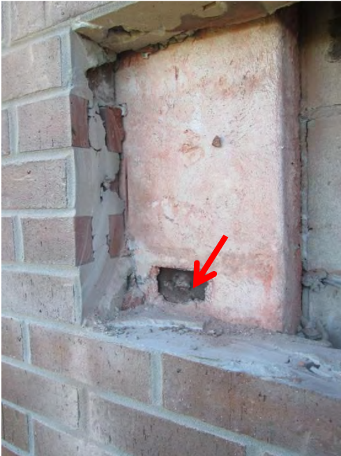
S35 - Missing welded wire tie at steel column backup
