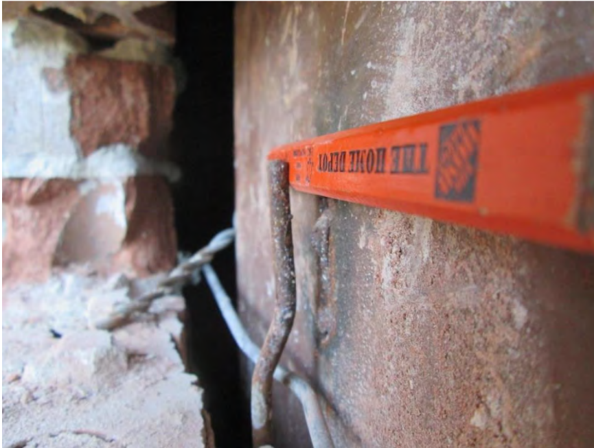
S37 - Broken weld at tie loop for brick tie connection shown in Photo 36
