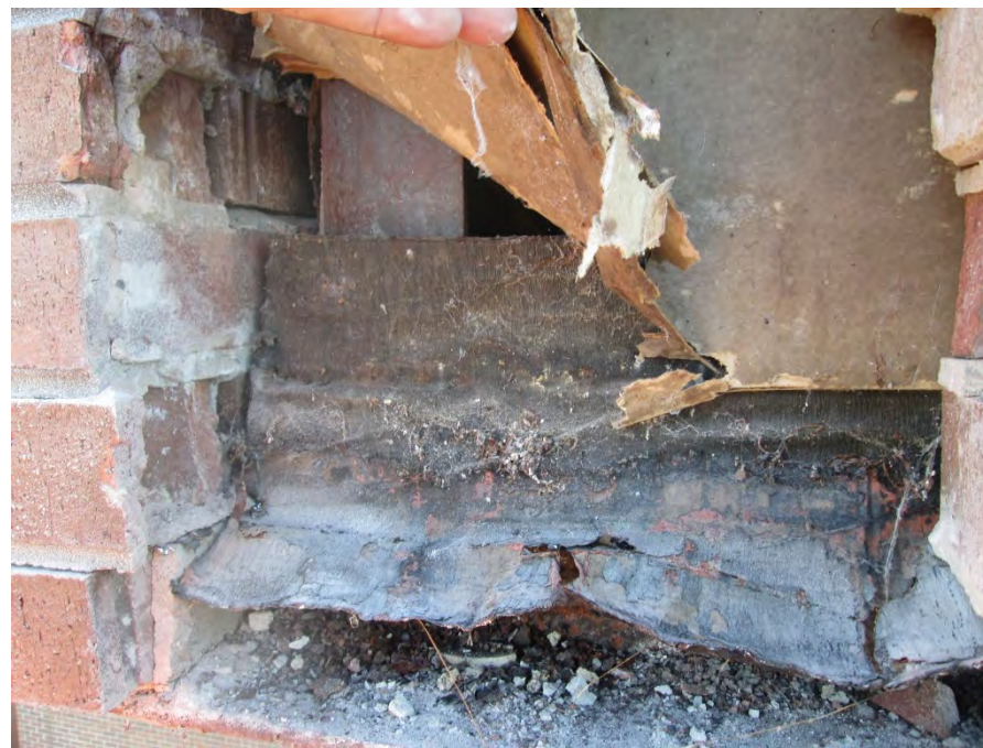
Discontinuous flashing of cavity wall waterproofing
