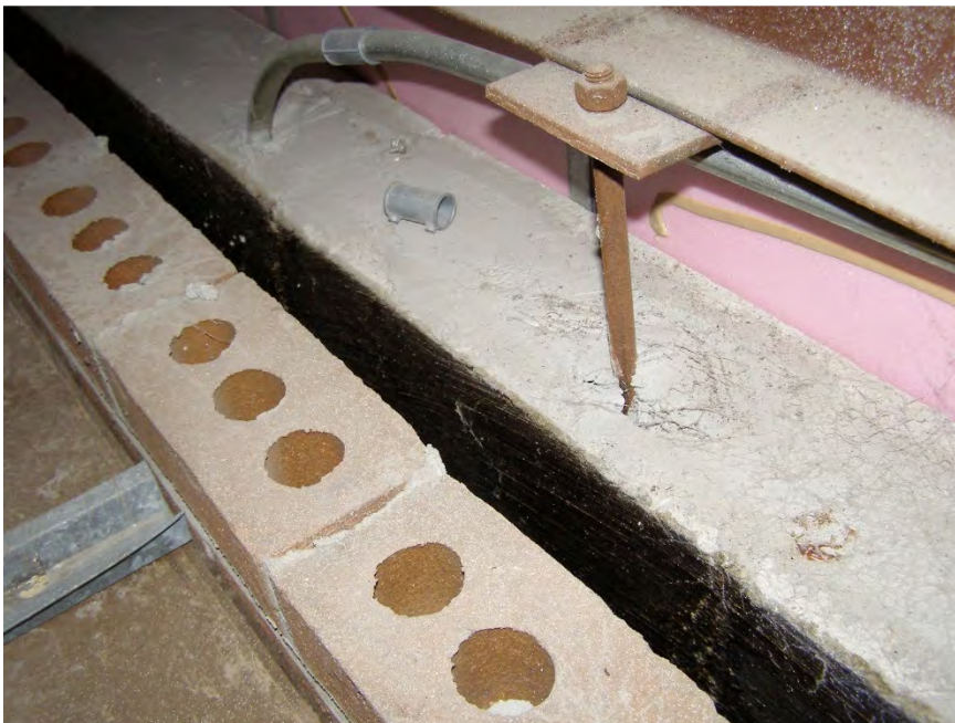
S76 - Top of inset wall at Level 3 on south side of building (top course of 6-inch CMU backup wall is grouted, photo shows anchor rod connected to bottom chord of joist and embedded in wall)
