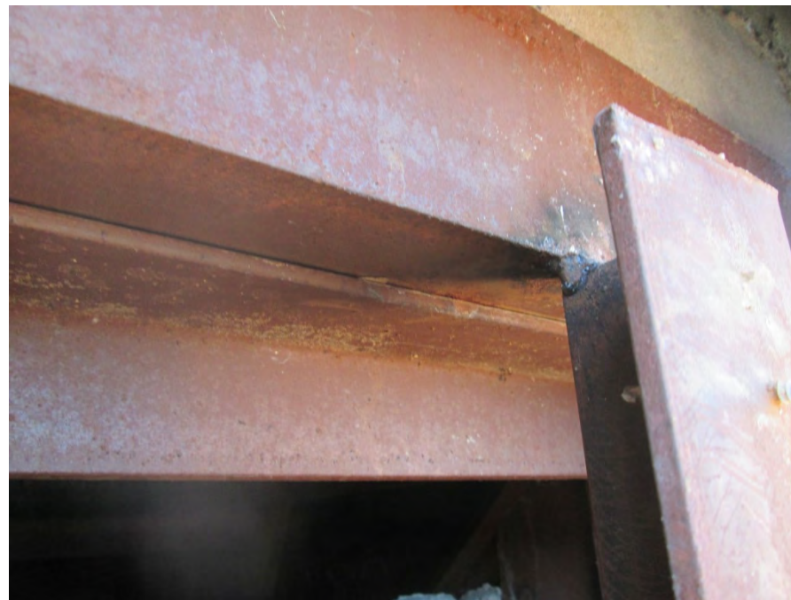
Tack welding of vertical angle support to metal deck closure angle
