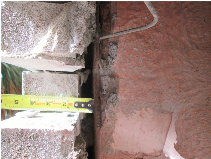
Wall cavity depth measured as 1-inch on south elevation of opening
