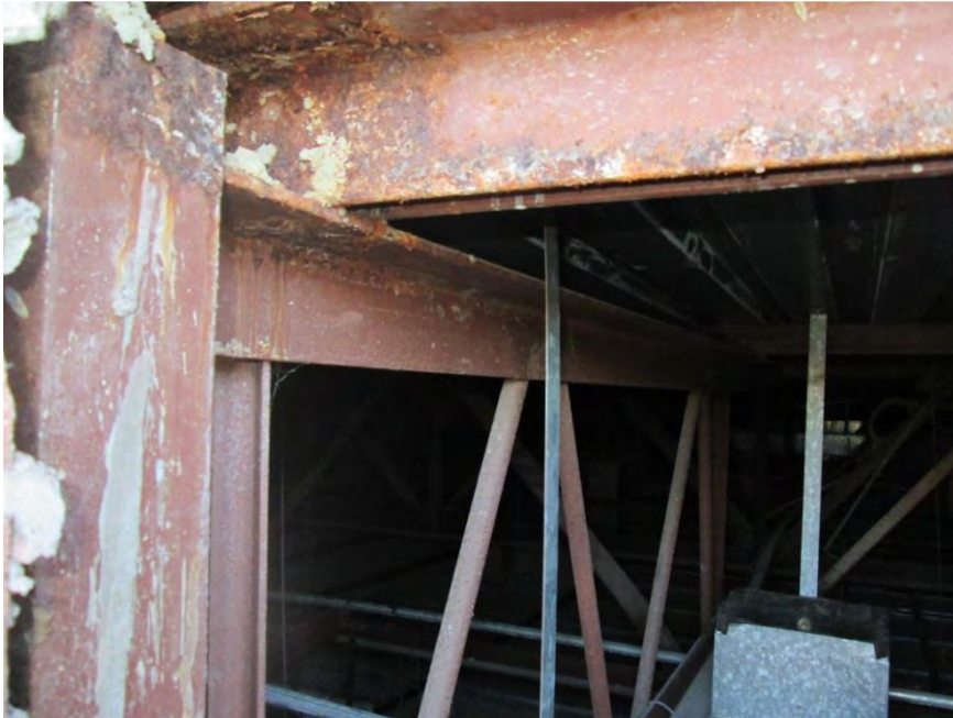
S27 - Corrosion of façade backup vertical steel and built-up joist bracing
