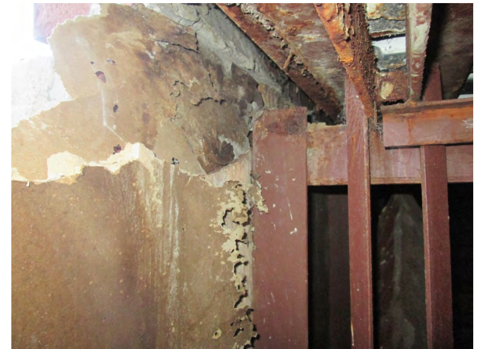
Corroded metal framing and deteriorated gypsum sheathing indicates previous water infiltration
