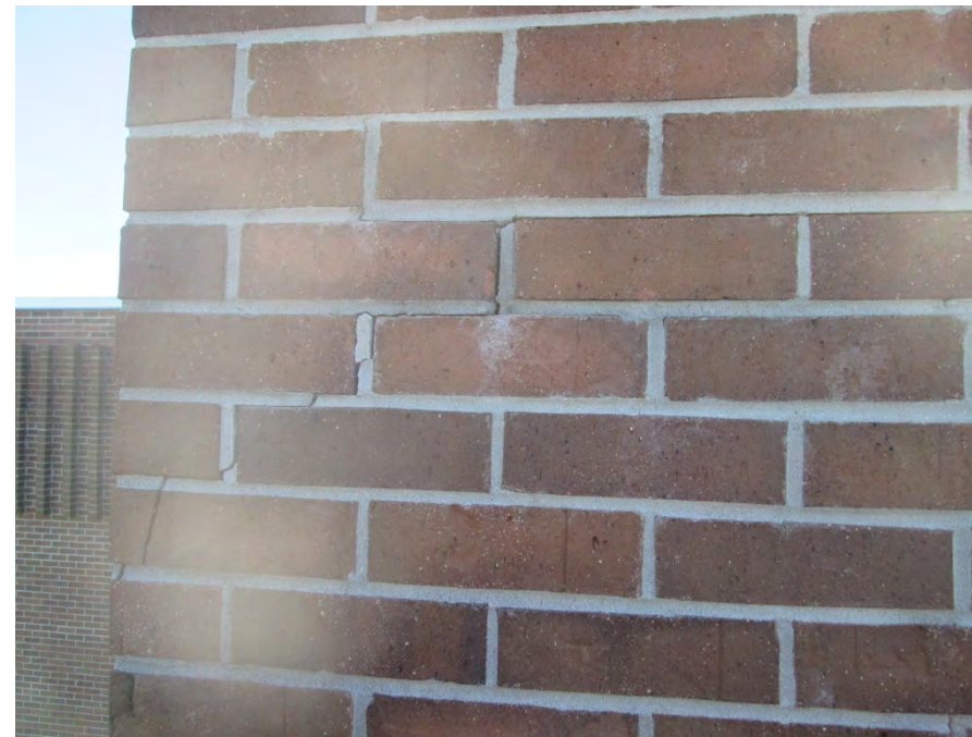
Brick cracking distress
