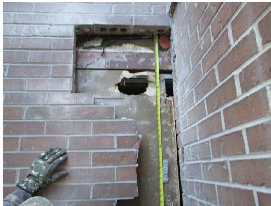
Vertical tie spacing measured at approximately 29-inches on center
