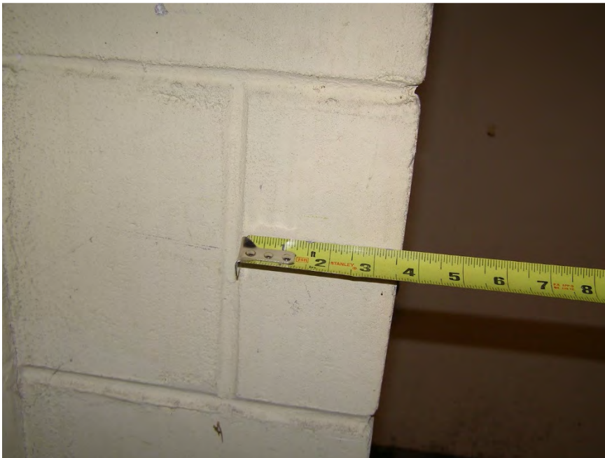
S80 - Tape measure shows width of nominal 4-inch CMU backup wall inside mechanical room
