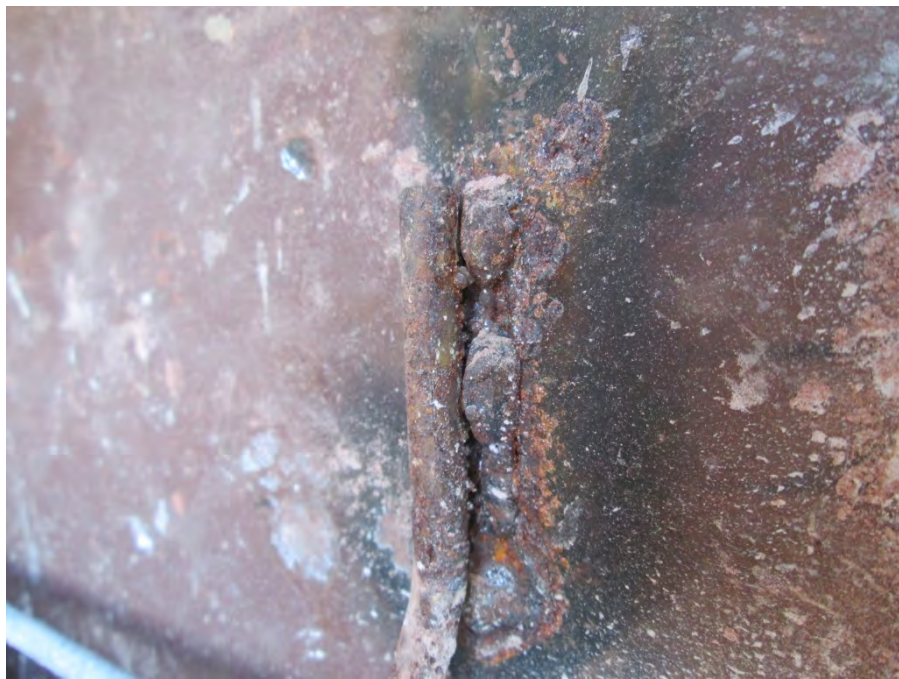
Corroded and broken weld at wire loop connection to steel tube column
