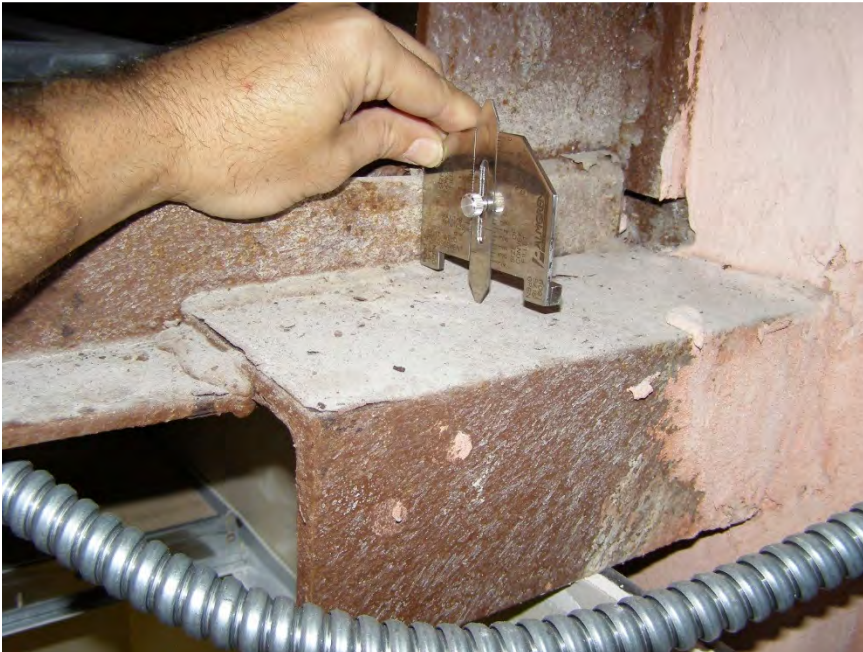
S62 - Close-up view of typical bottom chord-to-column moment connection consisting of angle welded to chord and column (photo also shows measurement of fillet weld)
