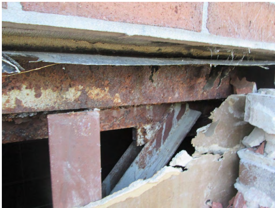
Corroded metal framing indicates previous water infiltration
