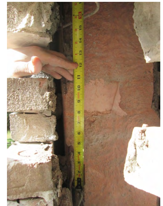
Vertical wire tie spacing measured as approximately 16-inches on center
