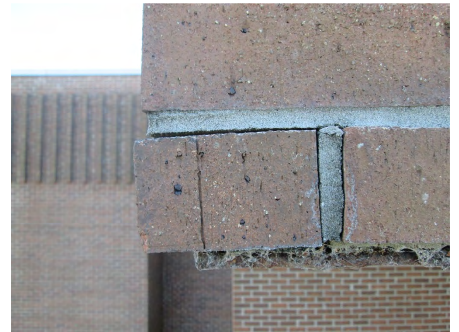
Rotated brick and mortar cracking at discontinuous shelf angle support
