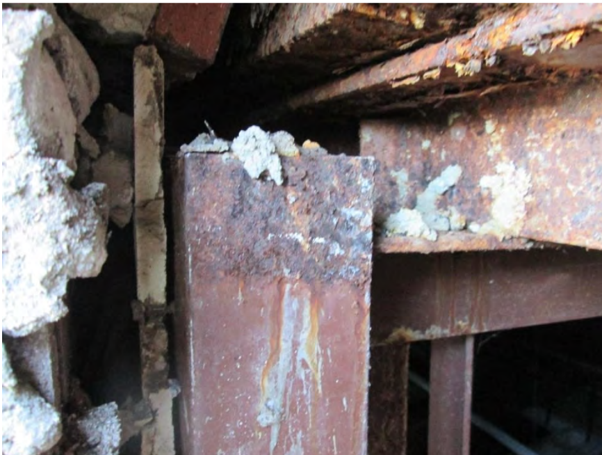
S28 - Corrosion of façade backup vertical steel and built-up joist bracing
