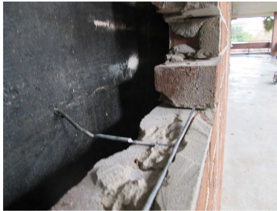
Ladder reinforcement embedded in brick masonry bed joint
