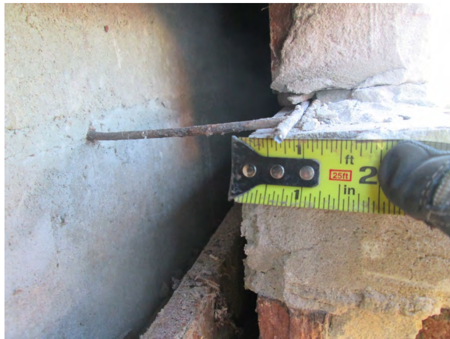
Ladder reinforcement tie not adequately embedded in brick masonry bed joint
