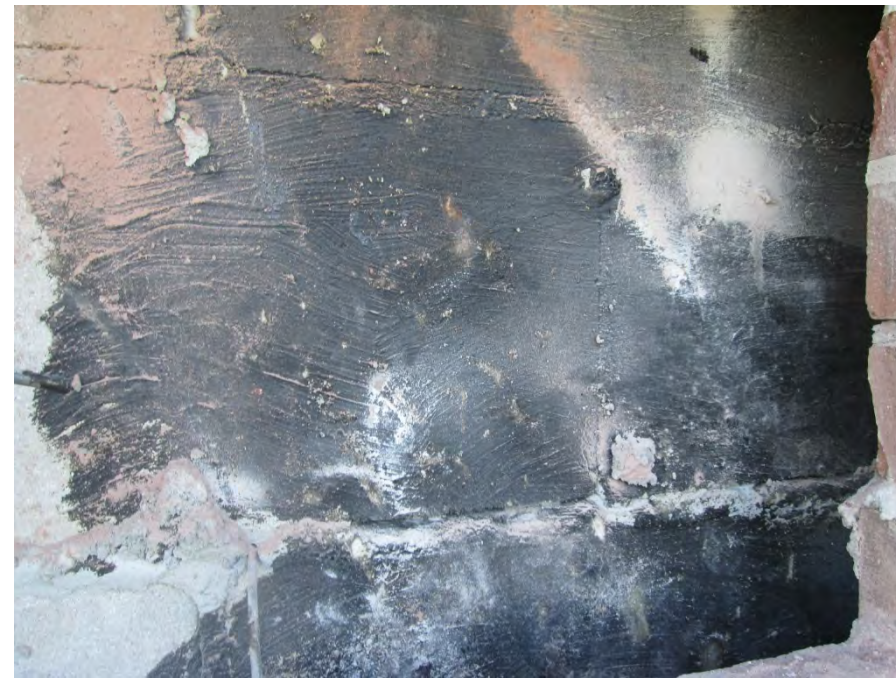
Fluid applied asphaltic waterproofing on CMU backup wall
