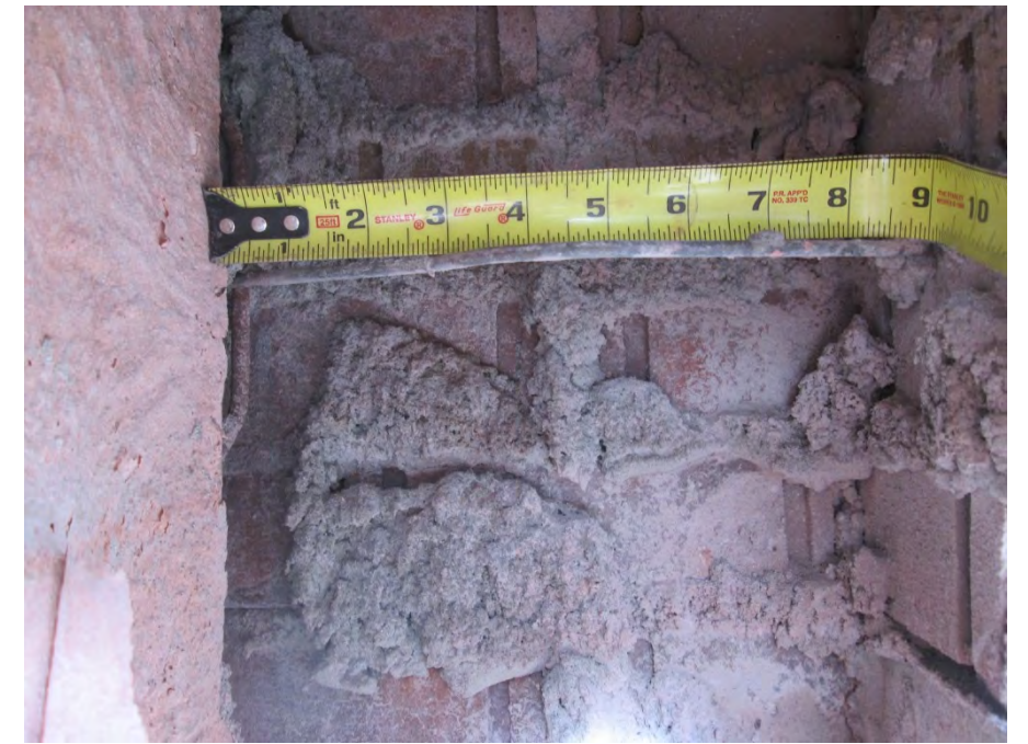
Wall cavity depth measured as 9-inches on west elevation of opening
