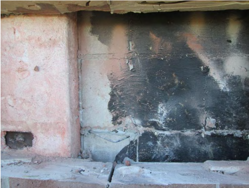
S31 - CMU wall backup system for façade cladding (noted fluid-applied dampproofing)
