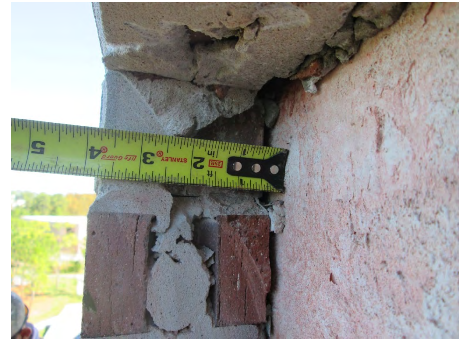
Cavity depth a steel tube column measured as 1/2-inch
