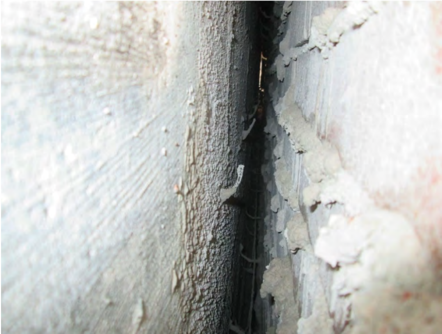
S41 - Cut section of horizontal ladder reinforcement spanning between Exploratory Openings 12 and 13
