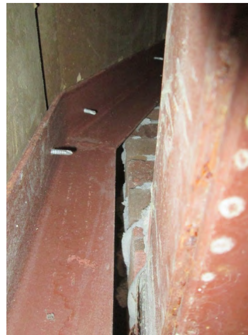
Bent steel angle backup for corbelled brick façade (view looking up towards start of corbelled wall section)
