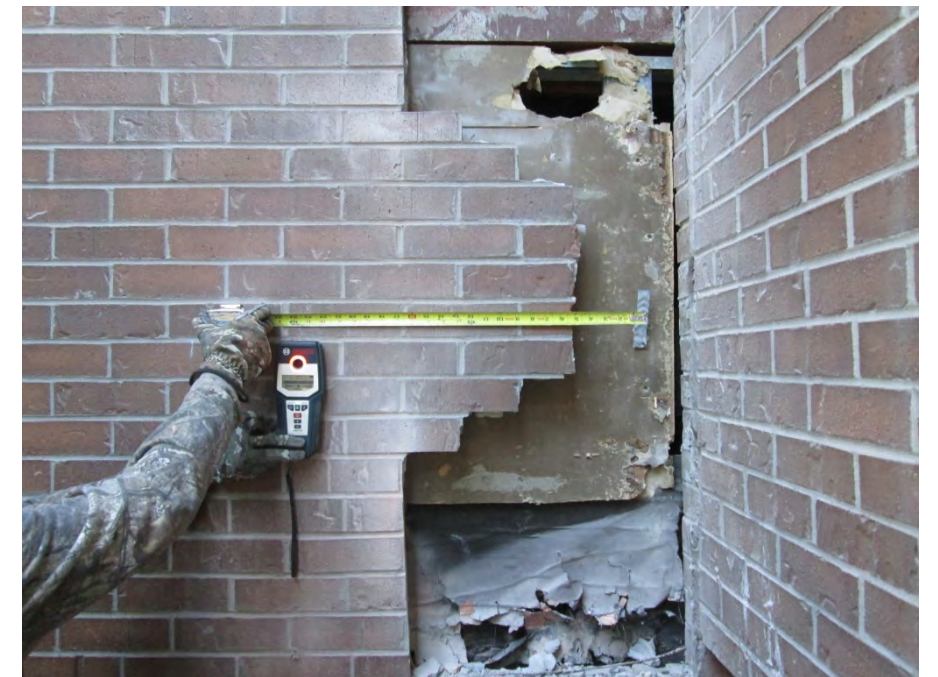
Horizontal tie spacing measured at approximately 24-inches on center
