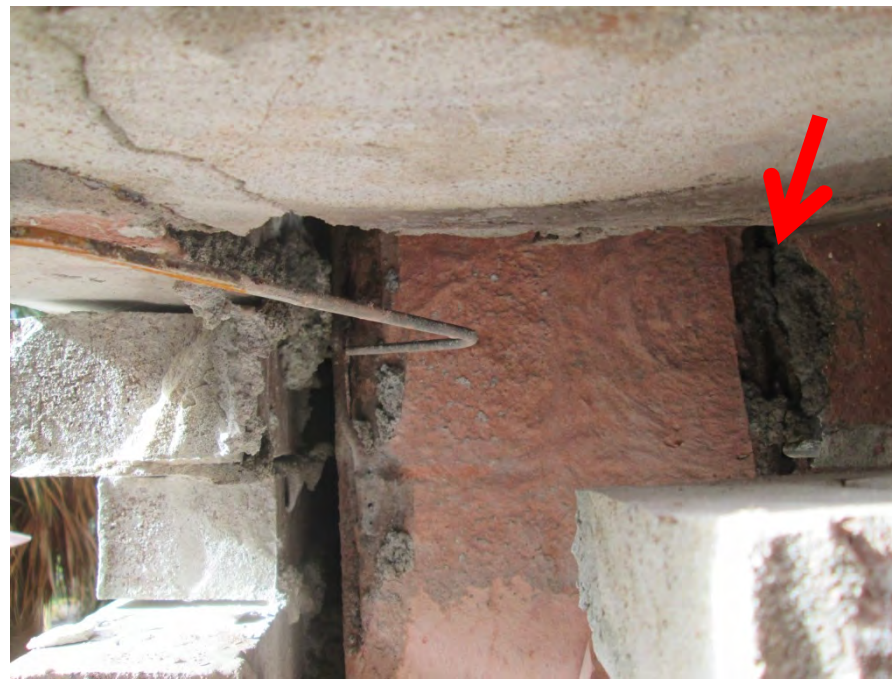
Mortar droppings at north elevation of opening inhibit cavity wall drainage
