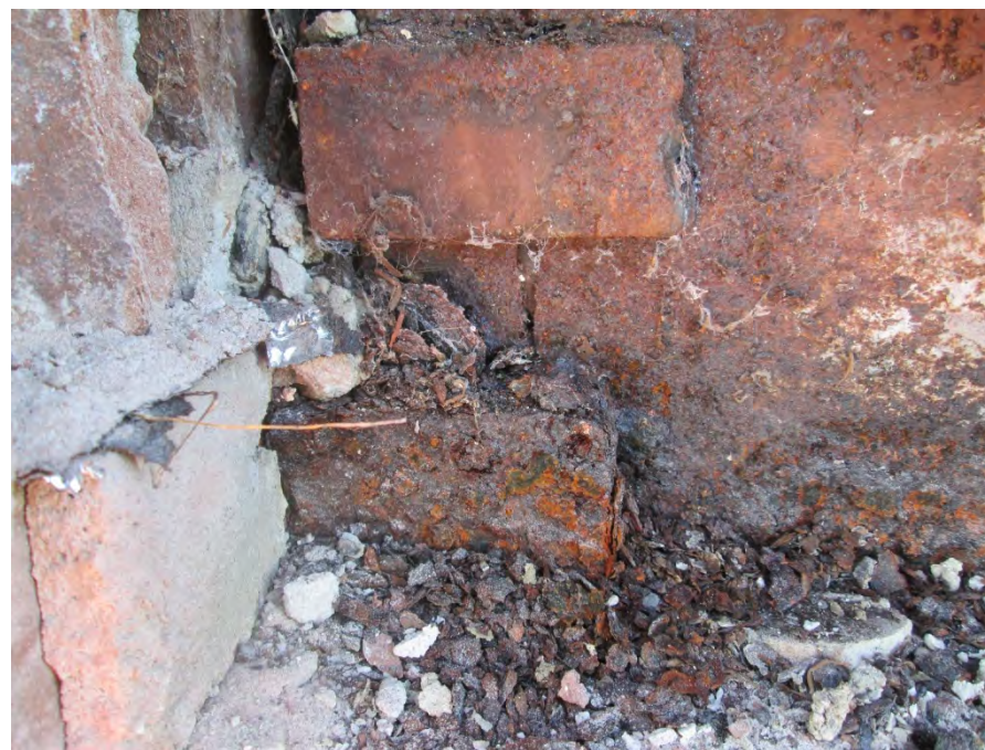
Corrosion distress at s discontinuous shelf angle splice connection
