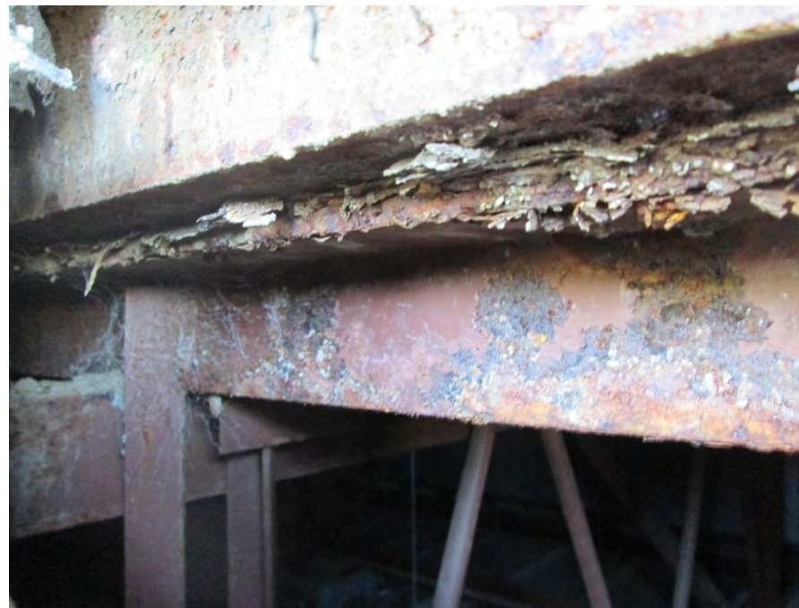
Corroded metal framing indicates previous water infiltration
