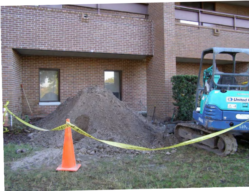
S50 - Excavation of exterior column footing on north side of building
