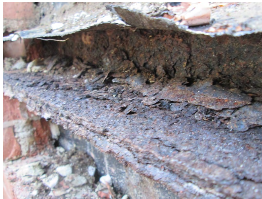
Corrosion distress at shelf angle
