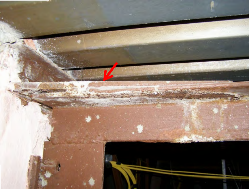
S63 - Close-up view of typical top chord-to-column moment connection consisting of angled plate (arrow) welded to chord and column
