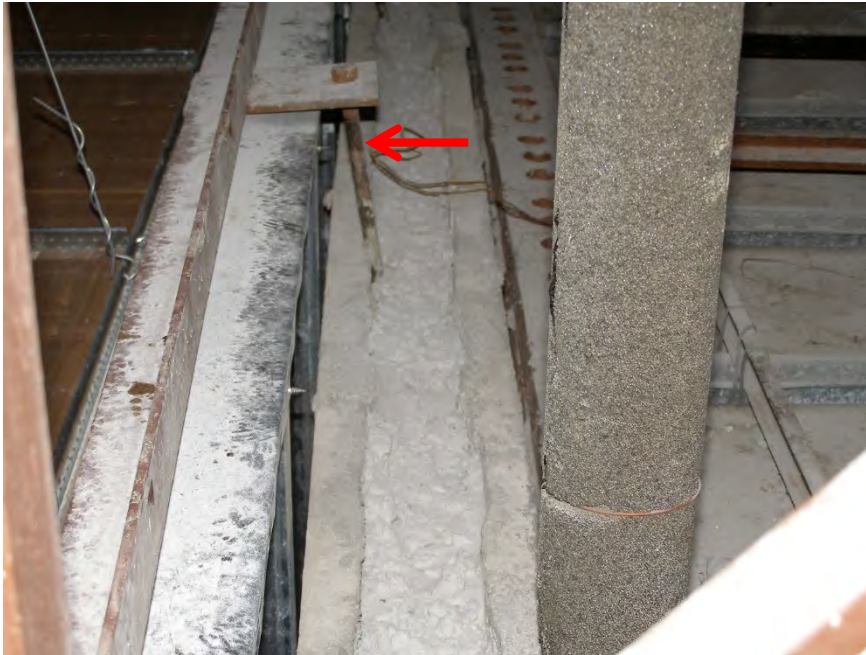
S75 - Top 6-inch CMU backup wall on south side of building below Level 2 exterior corridor (top course of masonry is grouted, anchor rod hung from joist above is embedded in wall)
