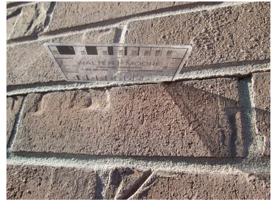
Brick crack width measured as 1/8-inch
