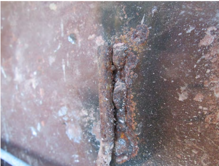
S36 - Corrosion noted at welded tie loop for brick tie connection
