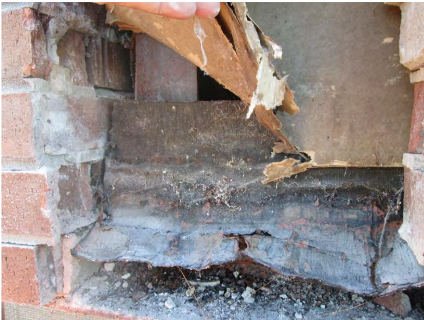
S48 - Discontinuous flashing waterproofing application at cavity wall
