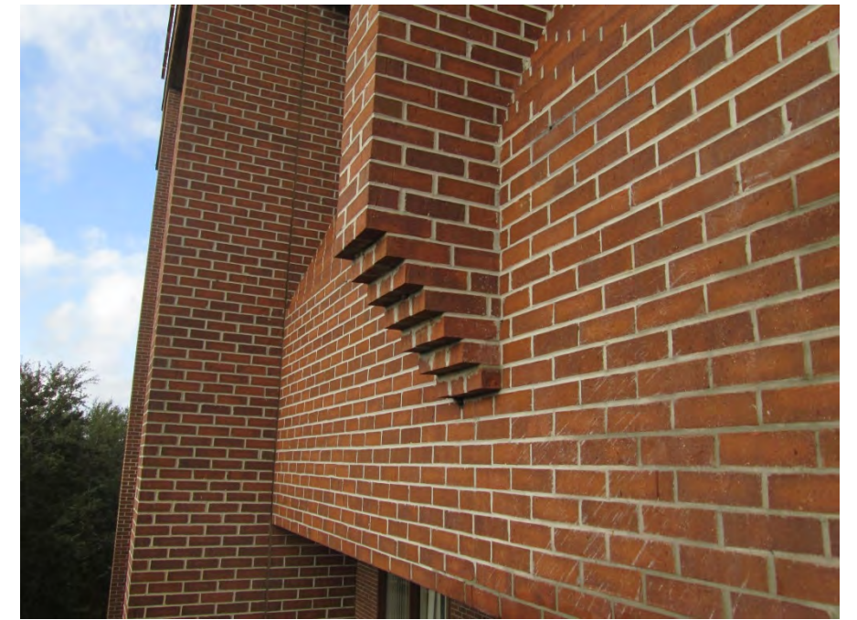
Corbelled brick façade at Level 4
