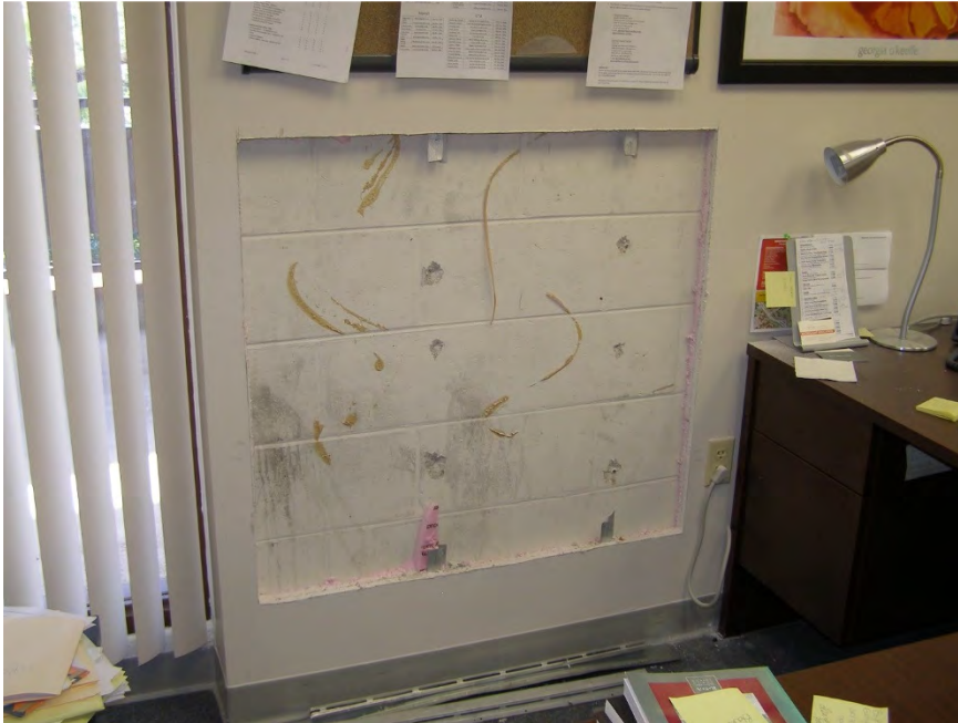
S77 - Typical opening in gypsum wallboard at interior face of setback exterior wall where GPR scanning was performed to check for the presence of vertical reinforcing steel
