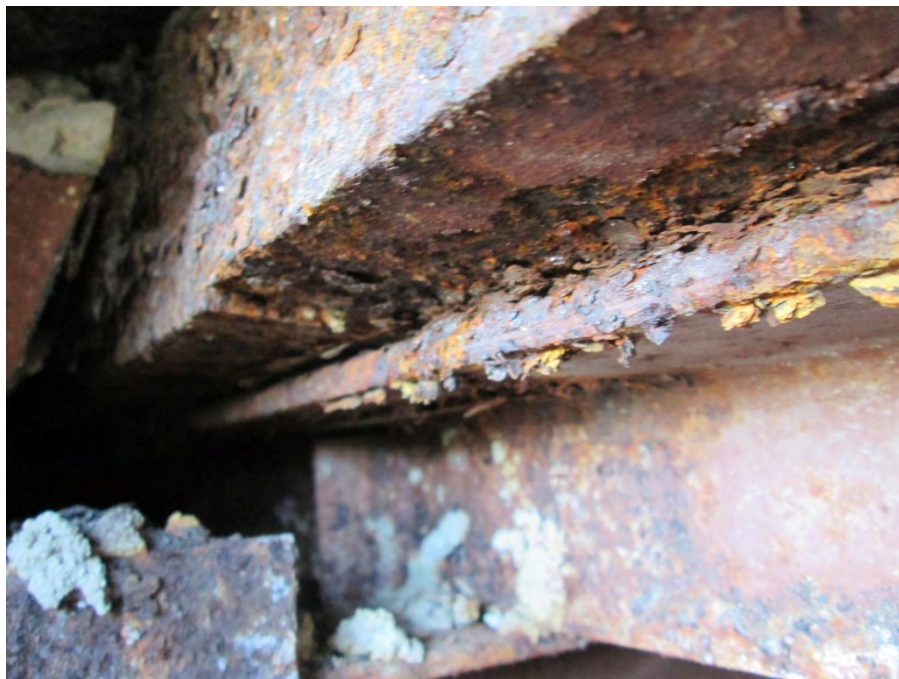
Corrosion distress at metal deck closure angle and joist girder top chord
