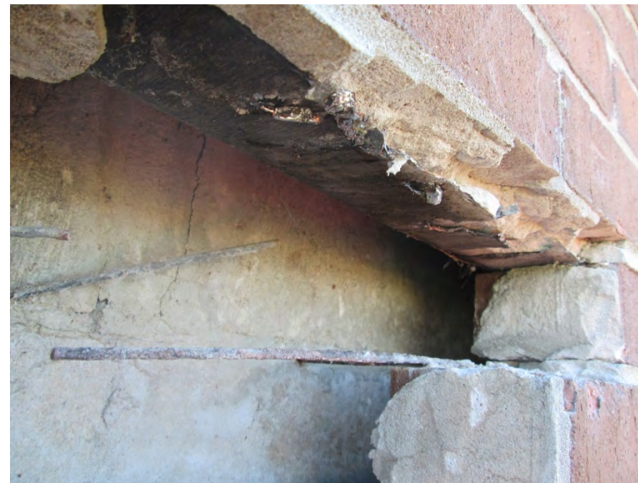
Through-wall fabric flashings act as bond-breaker for mortar joint
