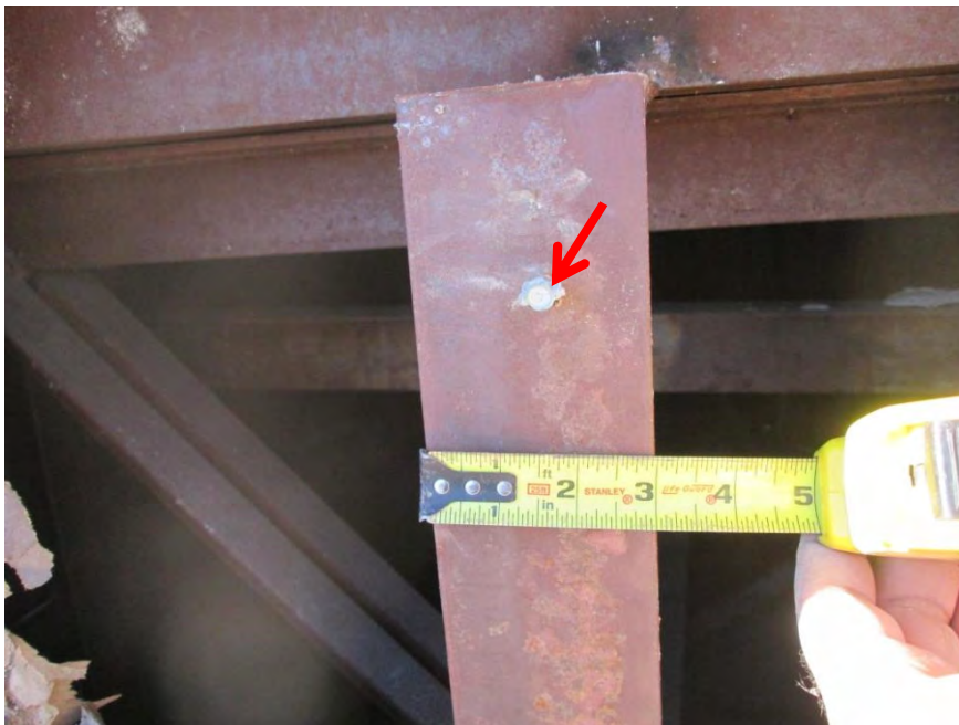
S34 - Missing corrugated brick tie at fastener to vertical steel angle backup
