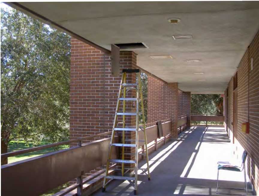
S64 - Soffit access panel used to access steel framing below exterior walkway on south side of Level 3
