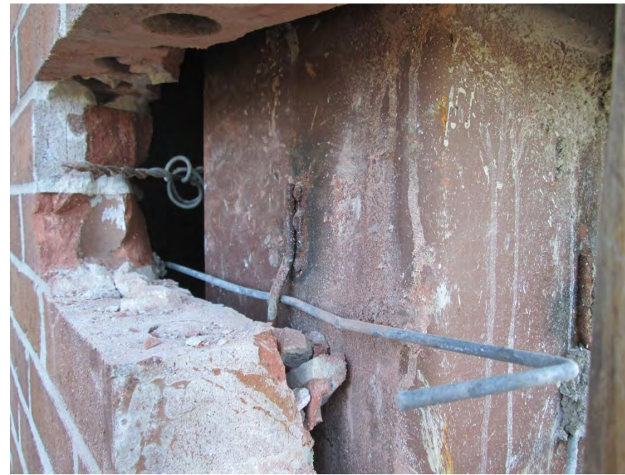
Wire tie attached to welded wire loops on steel tube column
