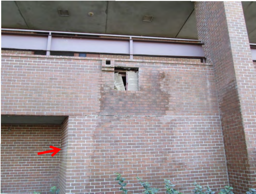
S73 - General view area of north elevation where observations of top of discontinuous CMU backup wall were made from façade exploratory opening (arrow highlights wall in following photo)
