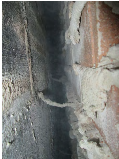
Ladder reinforcement attached to CMU wall backup
