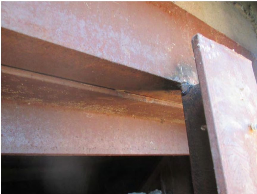
S26 - View of backup vertical steel angles tack welded to the metal deck steel closure angle
