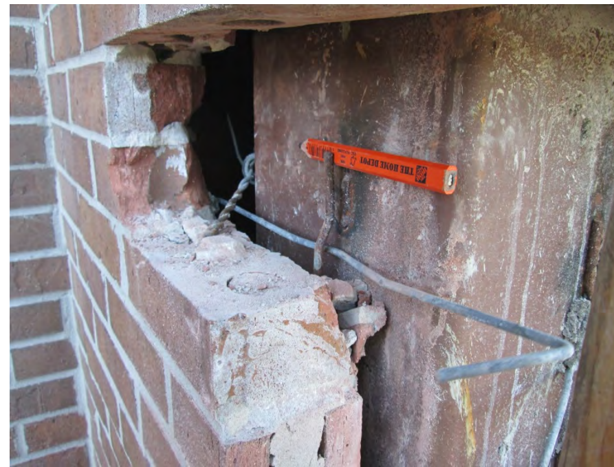
View of broken weld at wire loop connection to steel tube column
