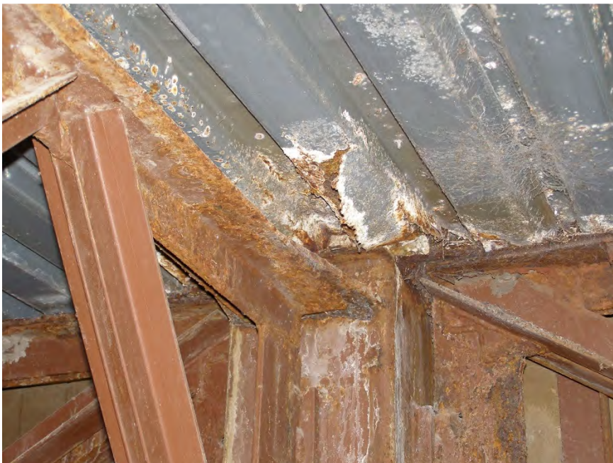
S68 - Closer view of corrosion shown in previous photo
