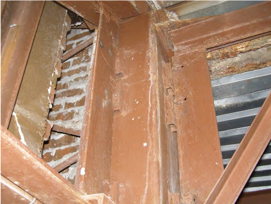
S65 - General view of area of long-term water intrusion at location shown in previous photo
