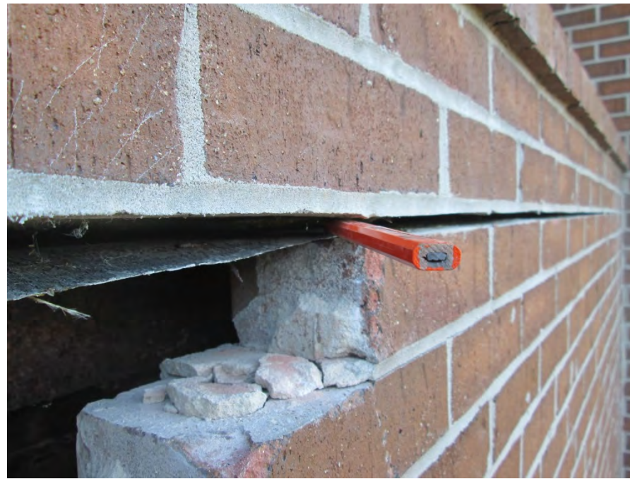
Deflected brick and separated mortar (through wall fabric flashing acts as bond breaker in masonry bed joint)
