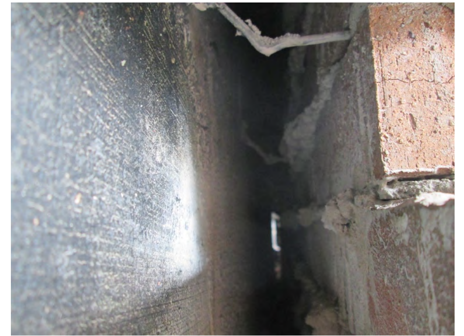
View of ladder reinforcement from CMU backup wall to brick masonry bed joint
