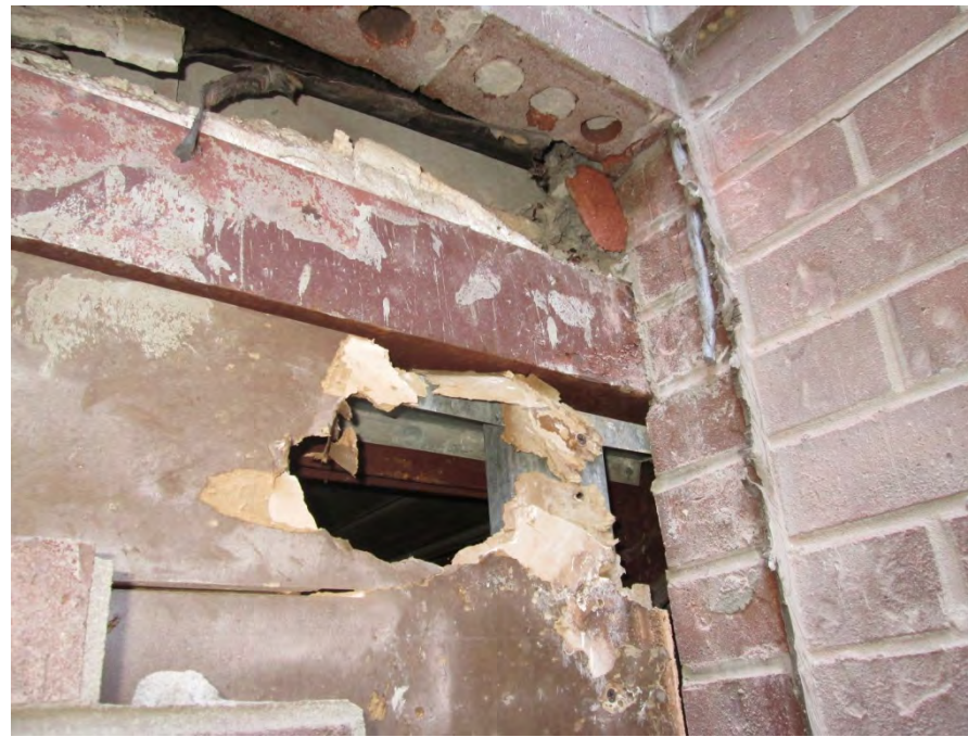
Metal stud with gypsum sheathing backup
