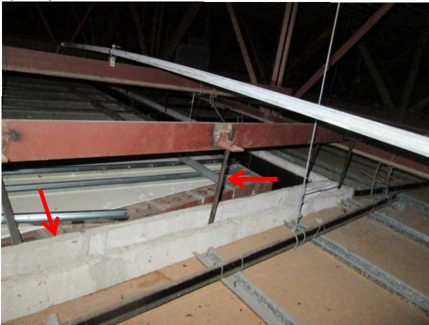
S74 - UngROUTED top course of CMU backup wall (left arrow), anchor rod hung from framing above highlighted by right arrow
