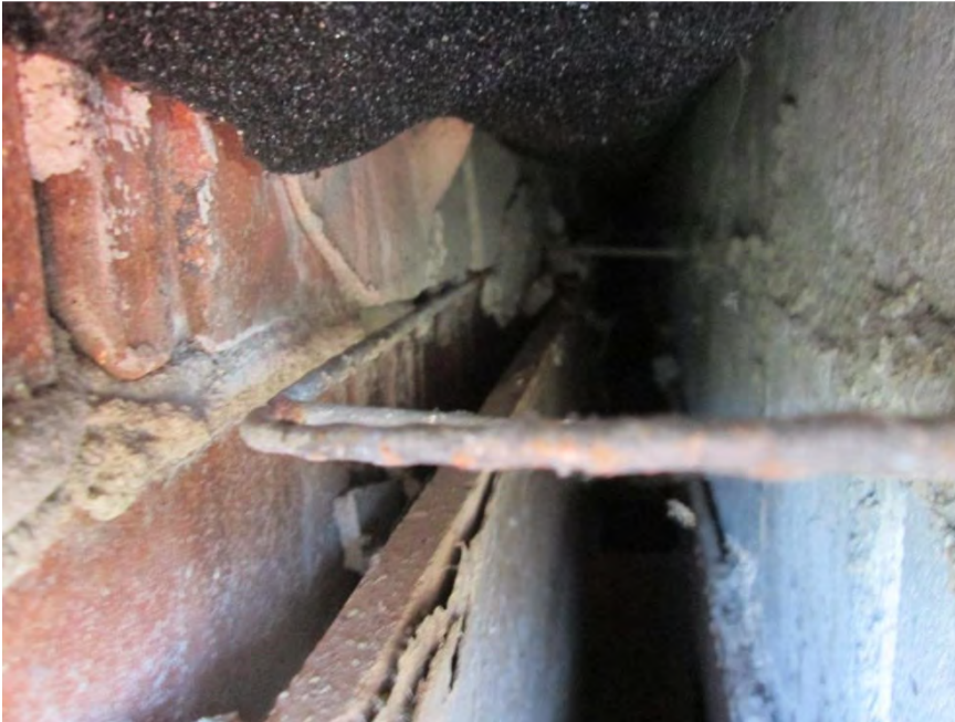
S39 - Horizontal ladder reinforcement not embedded in brick masonry bed joint
