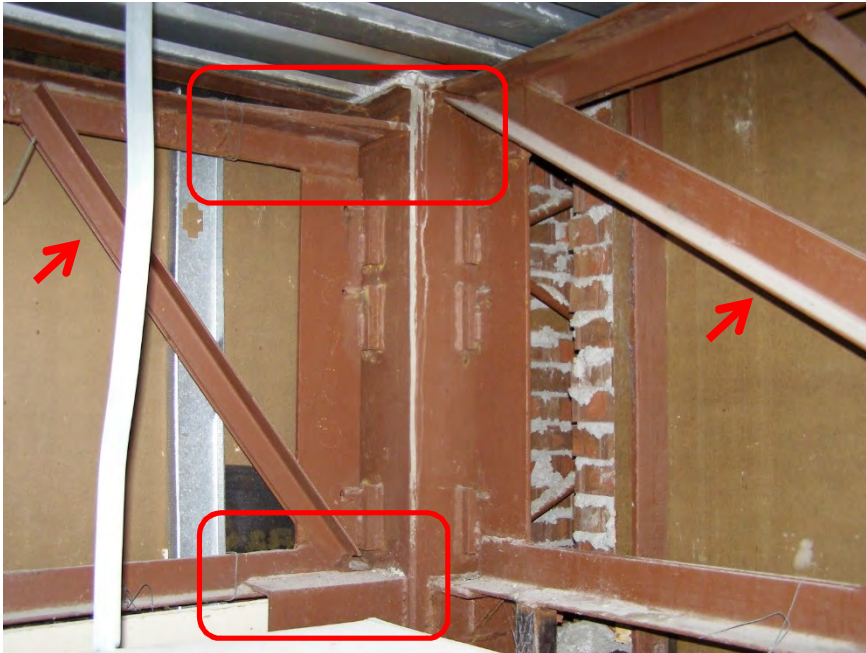
S61 - Typical joist/joist girder and column joint (joist girder highlighted by left arrow, joist highlighted by right arrow, lower box identifies typical bottom chord to column moment connection, upper box identifies typical top chord to column moment connection).
