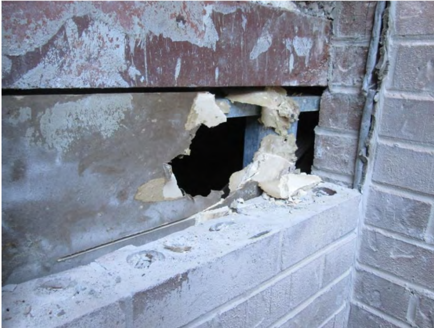
S29 - Metal stud and track framing for façade structural backup at attached tower structure
