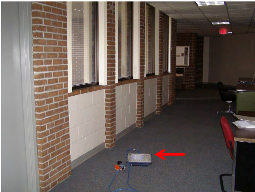
S78 - Exposed CMU backup wall at west end of Level 4 (arrow highlights GPR equipment)
