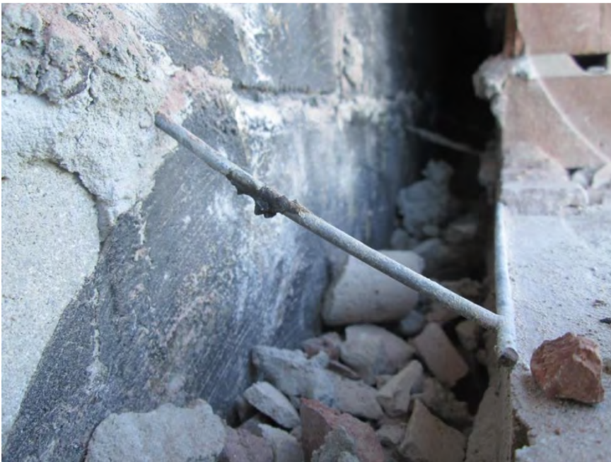
S40 - Horizontal ladder reinforcement not embedded in brick masonry bed joint (note ladder reinforcement is bent)
