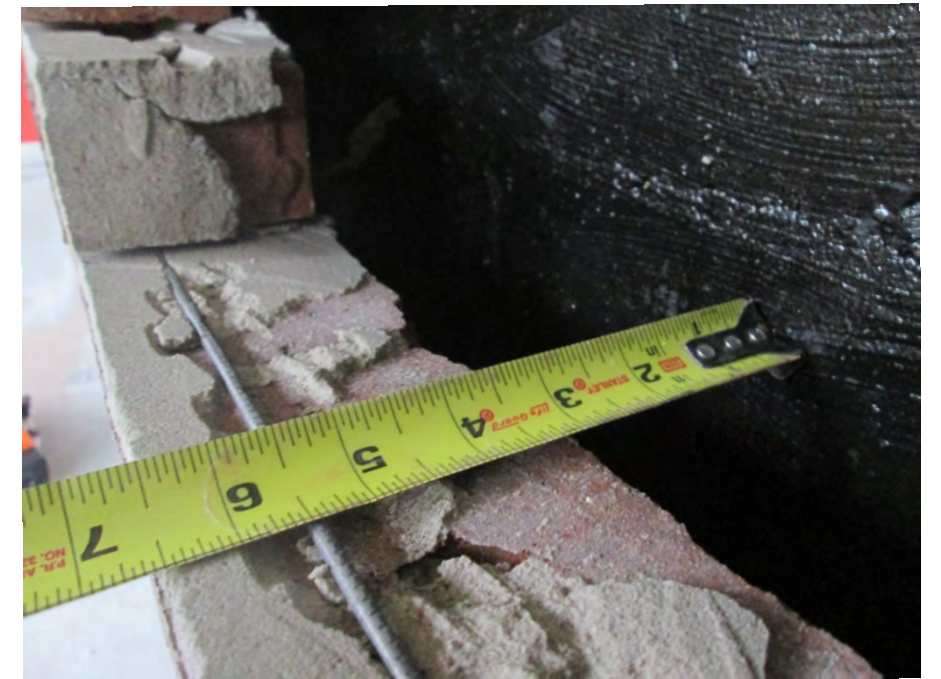
Ladder reinforcement embedded in brick masonry bed joint
