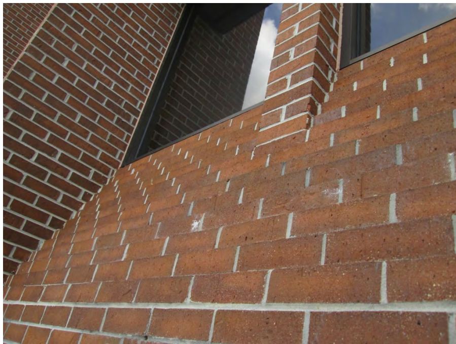
Corbelled brick façade at Level 4
