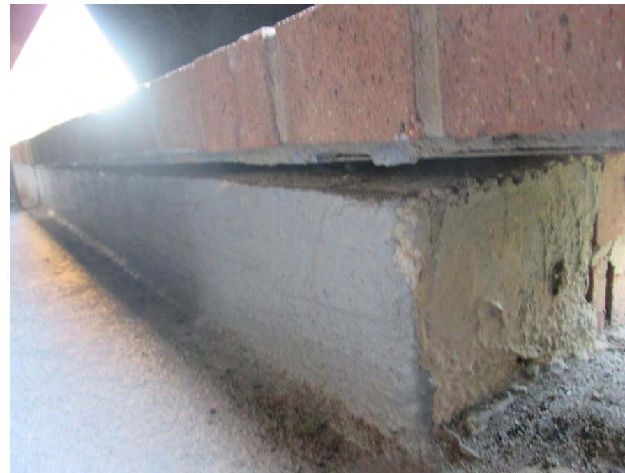
Gap between brick coping and concrete curb support (view from corridor)
