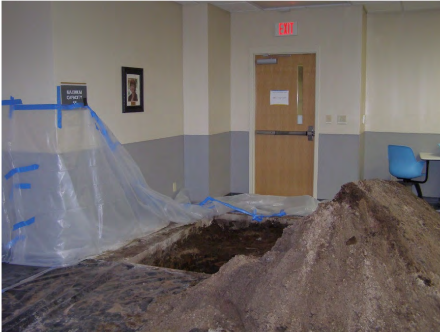
S53 - Interior column excavation
