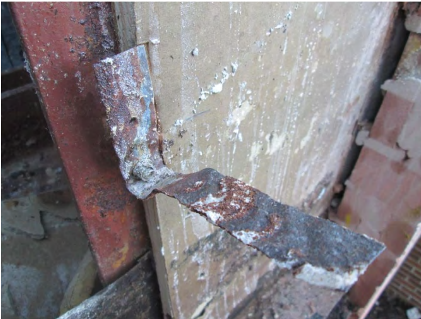
S32 - Corroded metal tie
