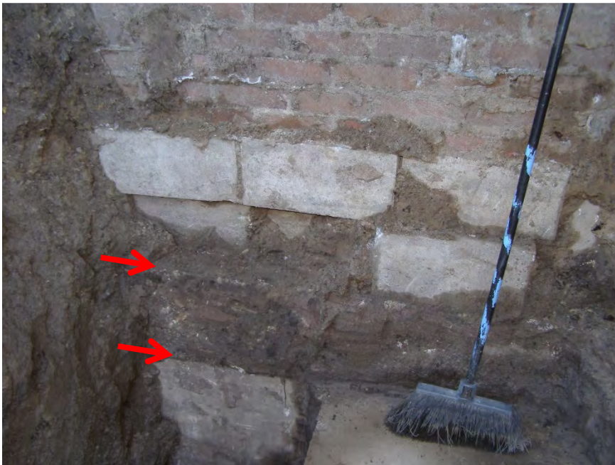
S52 - View of exterior wall at column footing excavation (lower arrow highlights top of interior column footing, upper arrow highlights continuous wall footing, concrete masonry units placed between wall footing and brick veneer).
