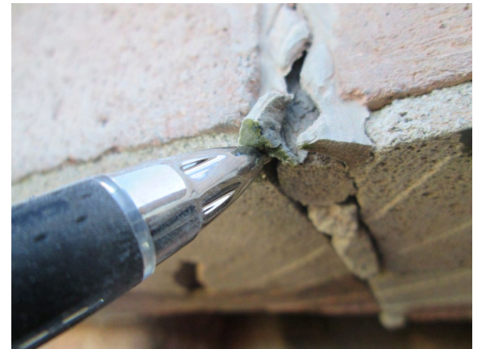
Joint sealant does not have an adequate width-to-depth profile ratio
