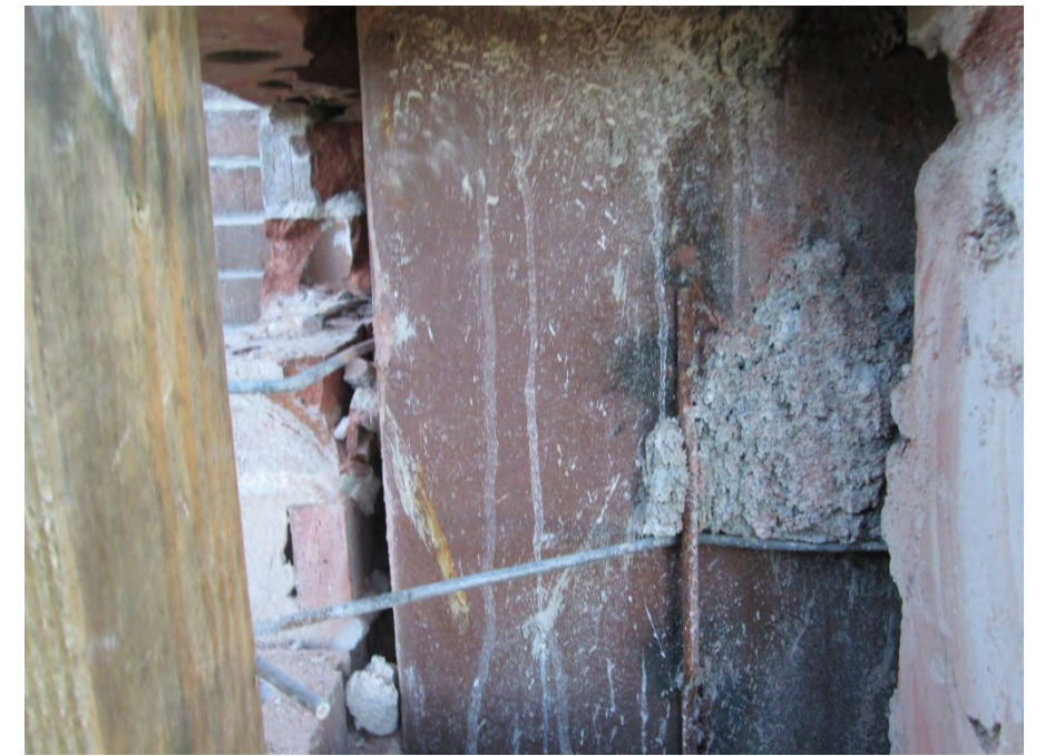
Wire tie attached to welded wire loops on steel tube column
