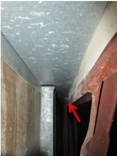
S30 - Cold-form metal stud and tracking framing (tracking attached to chords of spandrel joist)
