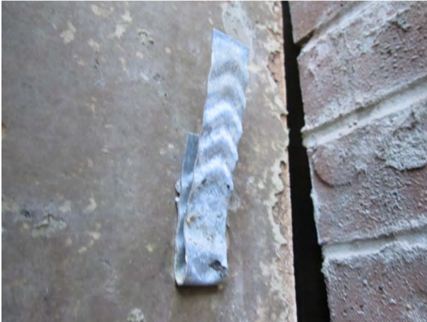
S33 - Corrugated metal tie not engaged in horizontal brick masonry bed joint (original construction condition)
