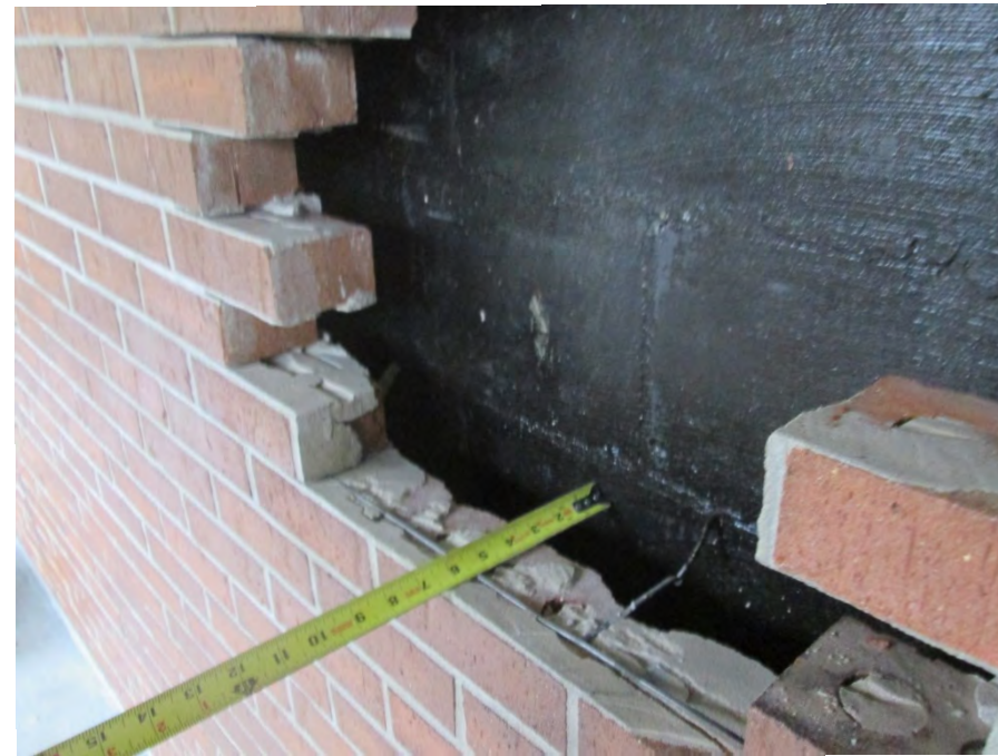
Ladder reinforcement embedded in brick masonry bed joint
