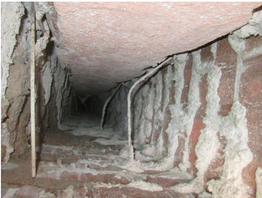
S38 - Wire ties attaching brick cladding to steel tube column at Exploratory Opening 10
