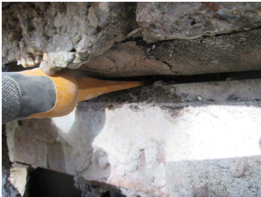
Gap between mortar bed joint for brick coping and concrete curb support
