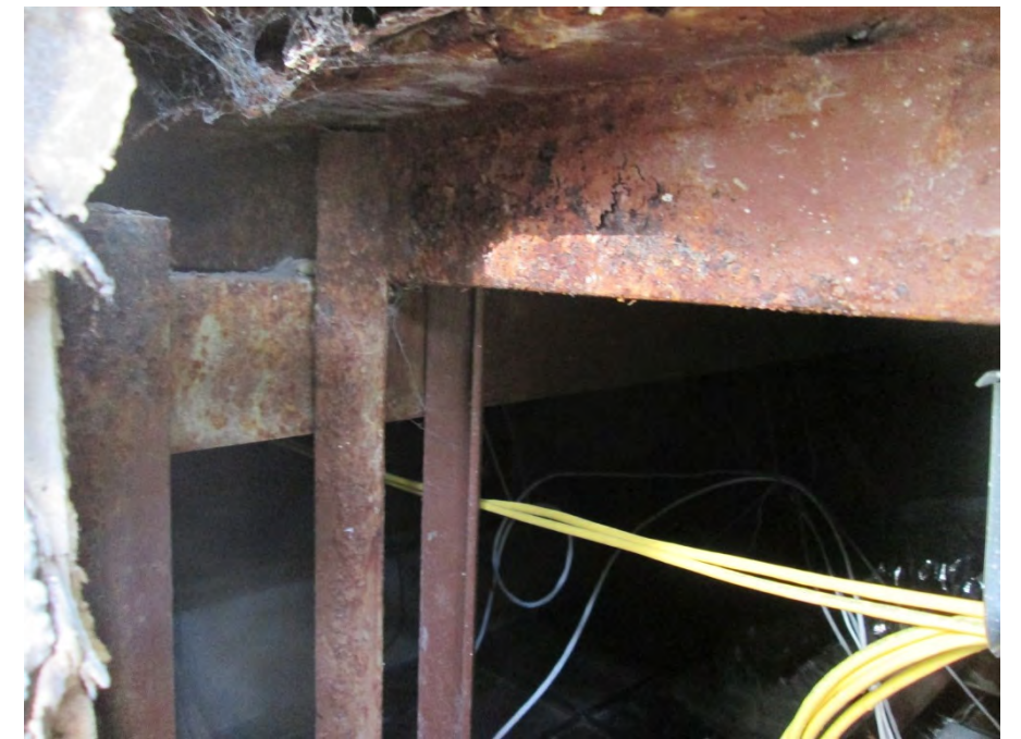
Corroded metal framing indicates previous water infiltration
