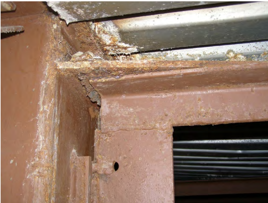
S66 - Close-up view of deck and structural steel corrosion shown in previous photo
