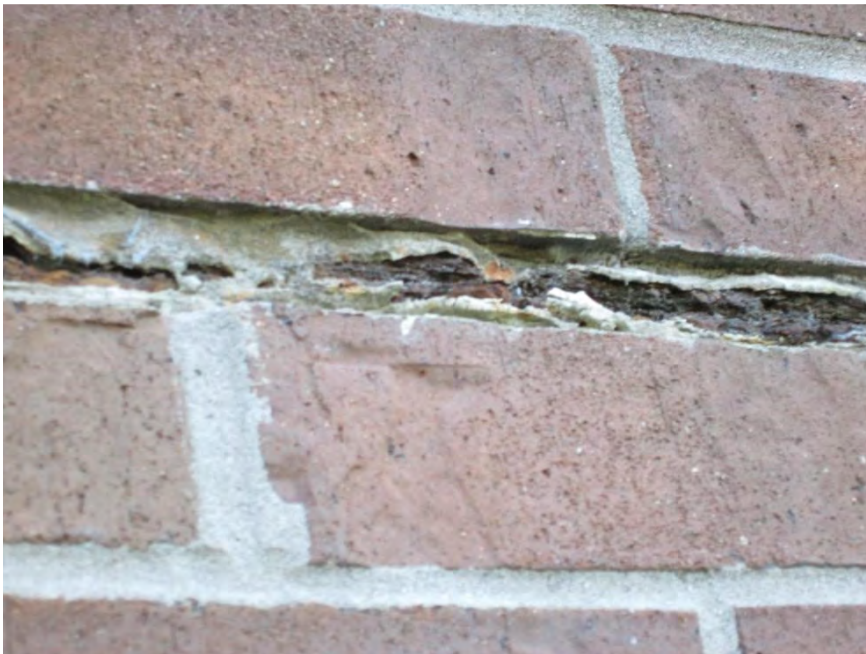
S18 - Corrosion at exposed shelf angle toe
