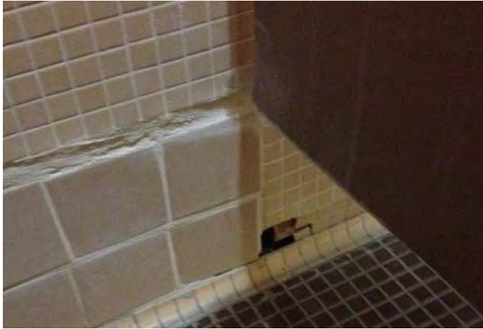
A19 – restroom, hole in wall, patch
