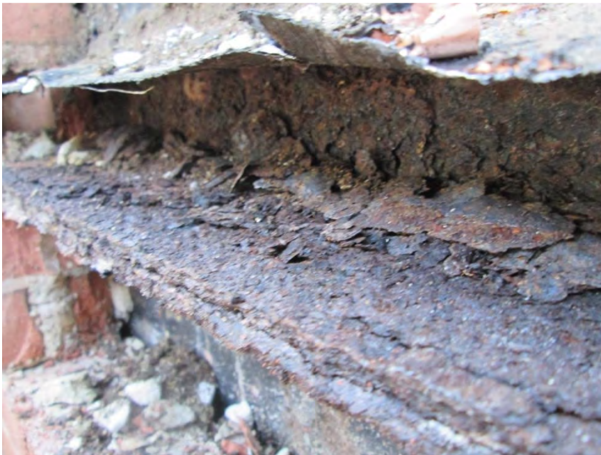
S20 - Close-up view of Photo 19 showing corrosion product buildup at shelf angle
