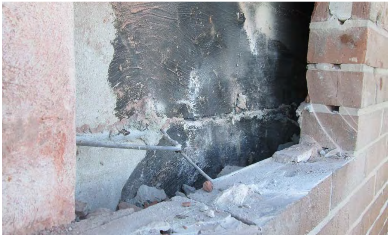
A3 – tower waterproofing lacking – cavity waterproofing coating, small air space, no insulation
