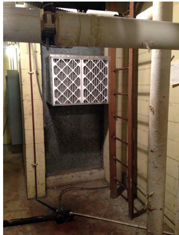
M2 – level 5 OA intake w/ no balancing
