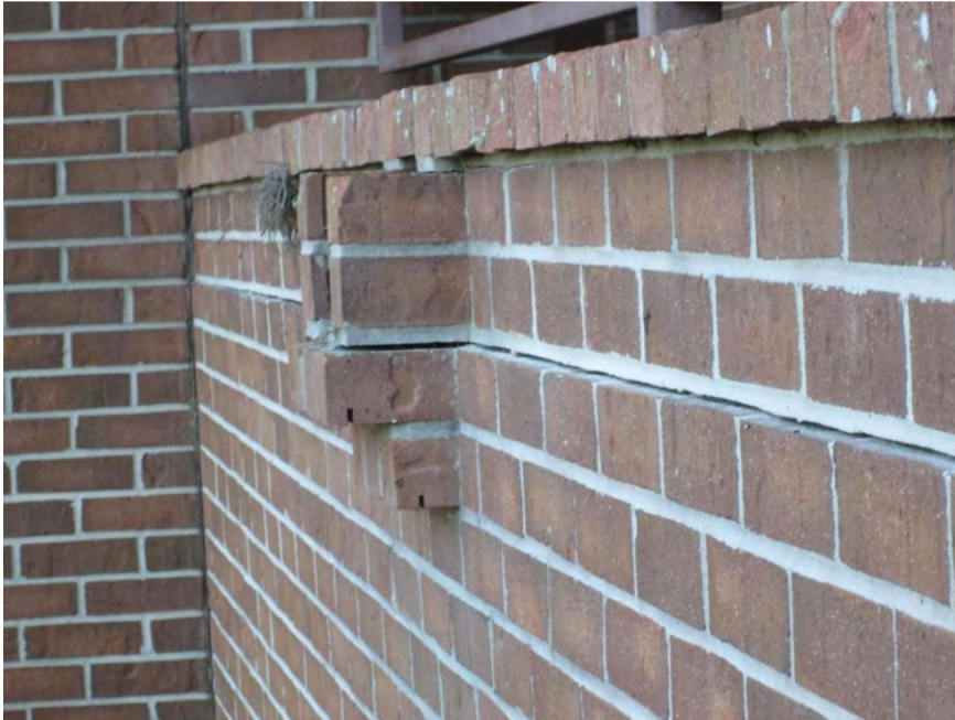
S7 – Separation at bed joint noted at top of Level 2 and Level 3 exterior corridor façade areas
