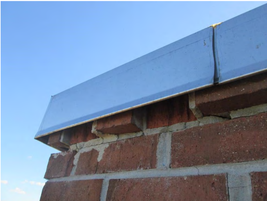
S2 - Close-up view of Photo S1 showing missing overhead brick below parapet wall coping
