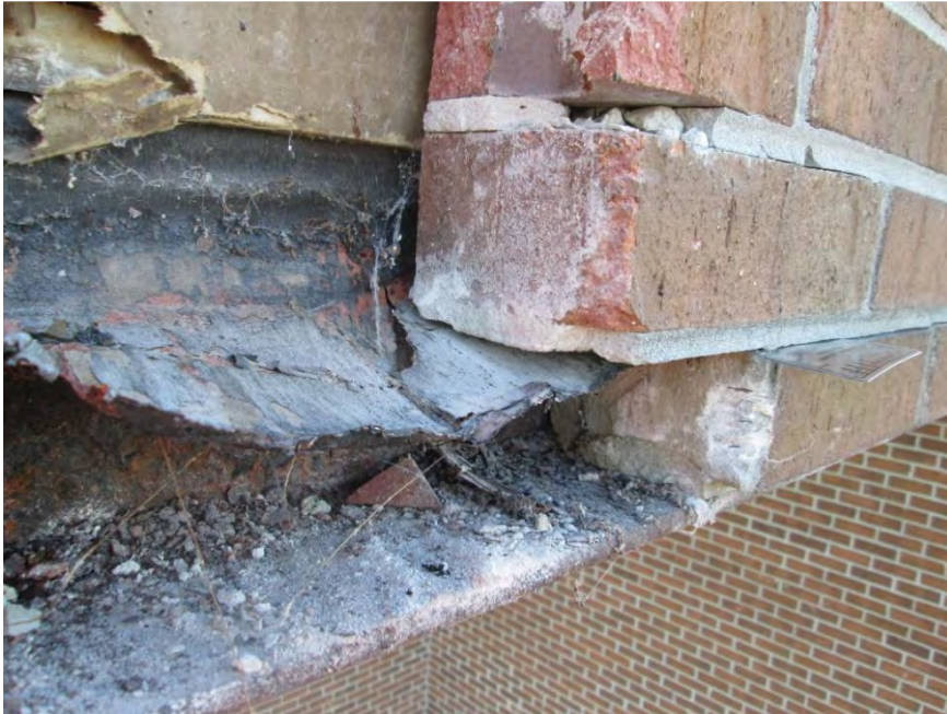
S17 - Mortar separation at brick courses below Roof Level parapet (note through-wall flashing)
