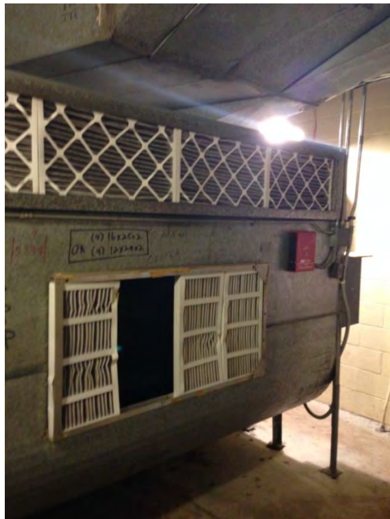
M3 – level 5 AHU return air opening
