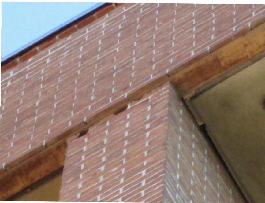
S12 - Spalled brick below shelf angle
