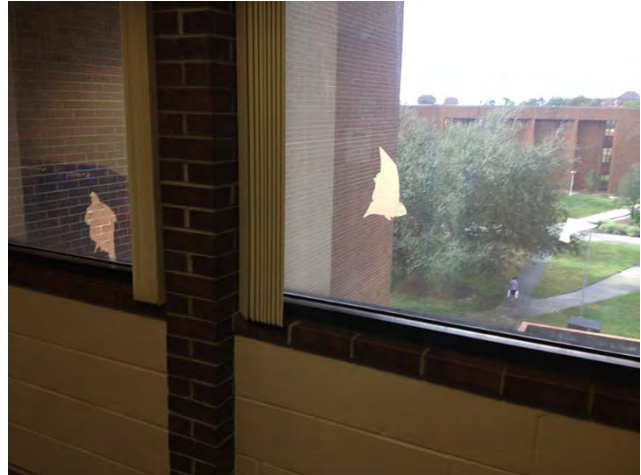
A12 – window film peeling, needs replacement
