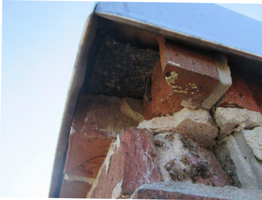
S5 - Disengaged fastener for parapet coping nailer attachment at missing brick location
