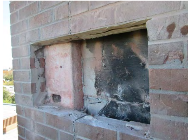
tower waterproofing – deteriorating and not consistently applied, no vapor barrier, no insulation
