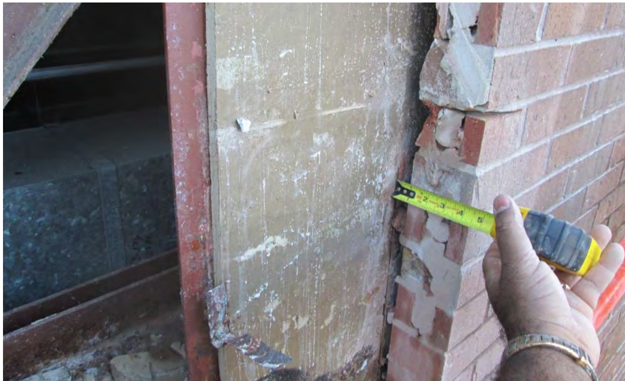
A6 – main building waterproofing lacking – gwb with no waterproof coating, small air space
