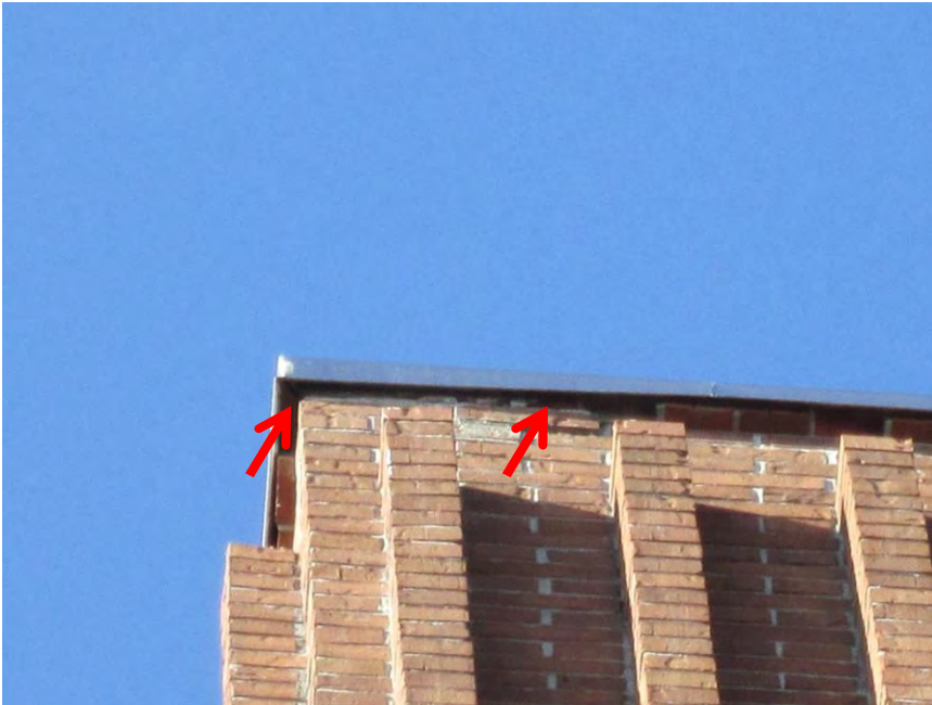
S1 – View of missing brick beneath Roof Level parapet wall coping cap
