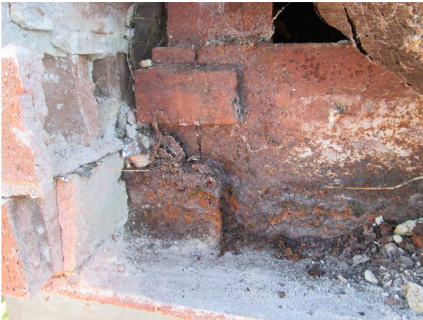
S24 - Spliced discontinuous shelf angle at Exploratory Opening 6
