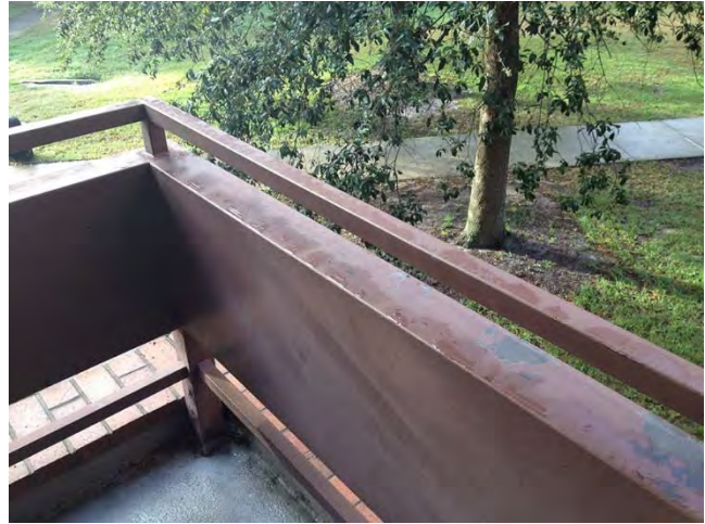
A16 – handrail standing water
