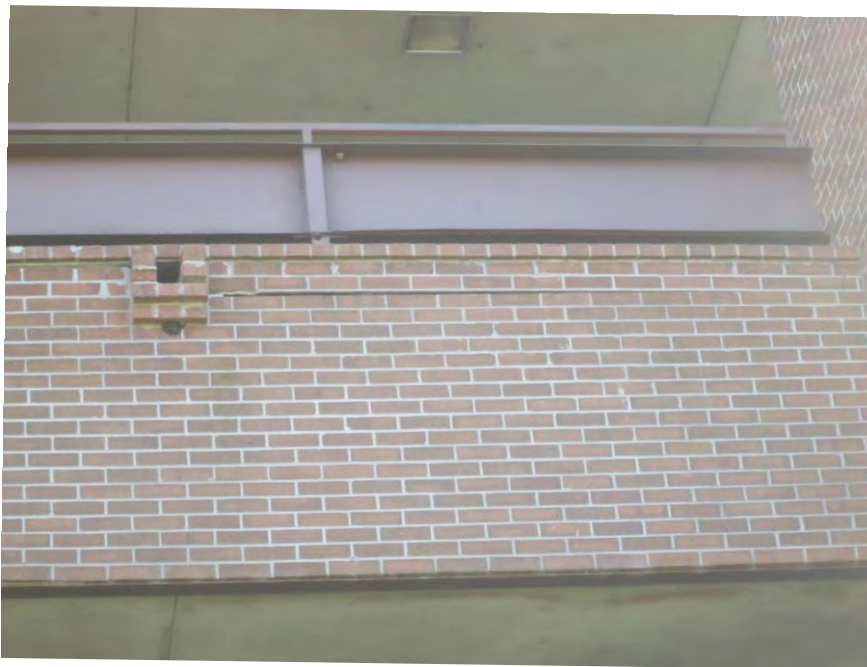
S6 – Separation along bed joint noted at top of Level 2 and Level 3 exterior corridor façade
