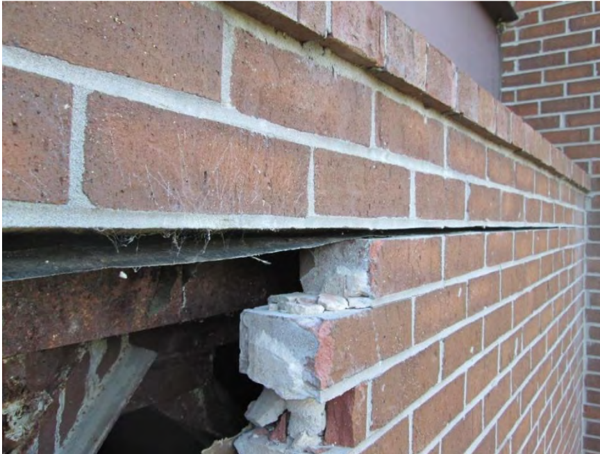
S15 - Mortar separation at exterior open corridor brick coping (note through-wall fabric flashing)
