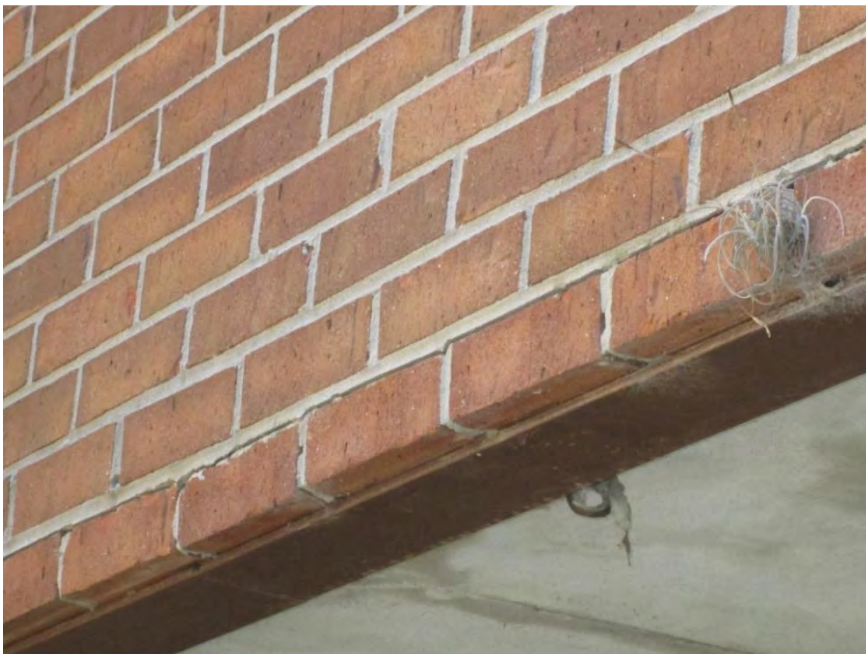
S8 - Potentially loose overhead brick at Level 2 exterior open corridor areas above Level 1 access walkways
