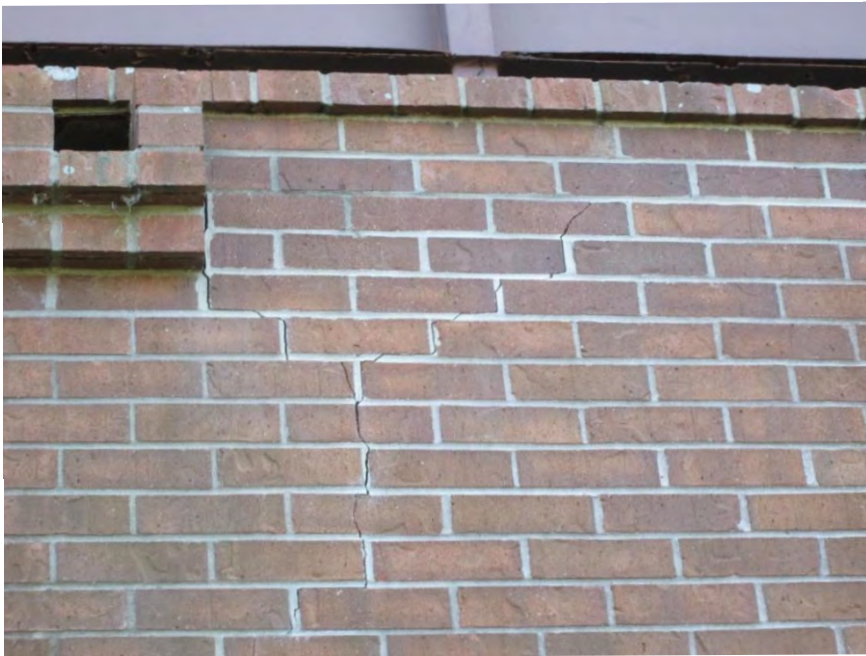
S9 - View of cracked brick
