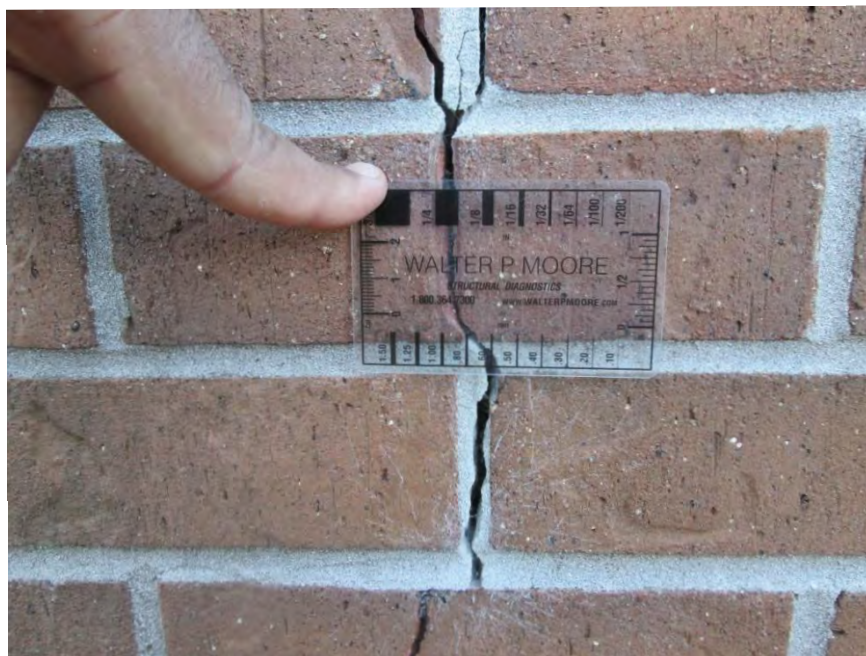
S10 - Close-up of Photo S9 showing 1/4-inch wide brick cracking
