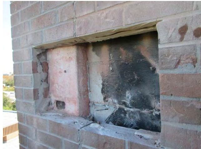
A2 – tower waterproofing lacking
