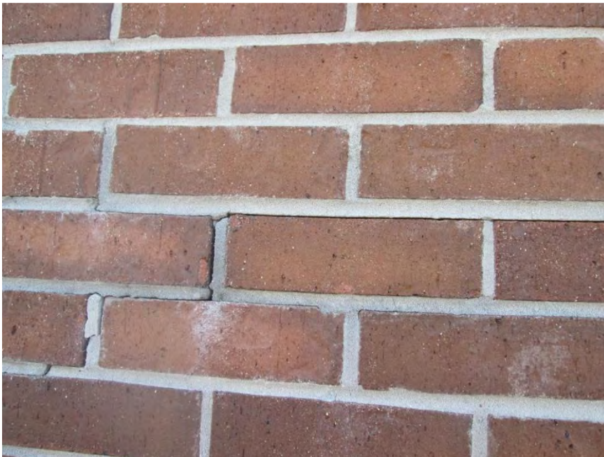
S14 - Brick mortar cracking
