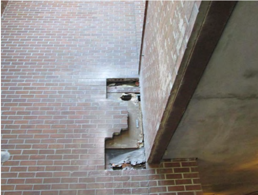
S23 - Shelf angles not noted in exploratory opening at attached tower structure
