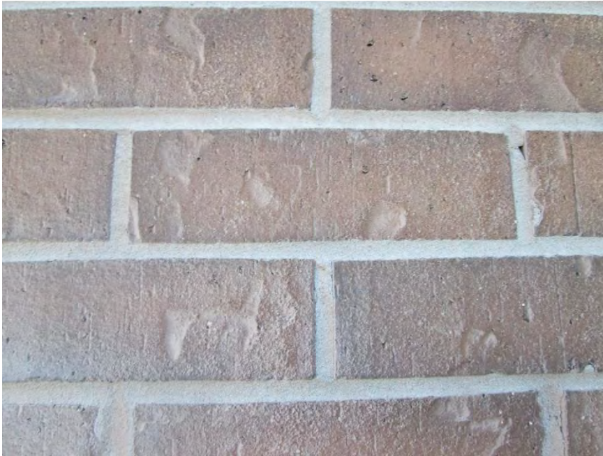
S13 - Mortar joints generally noted to be in fair condition
