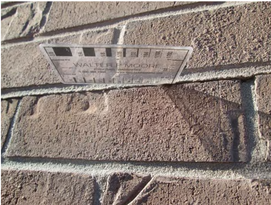
S16 - Mortar separation at brick courses below Roof Level parapet
