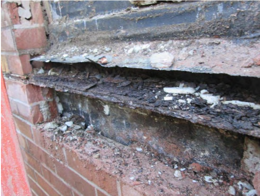
S19 - Corrosion product buildup at shelf angle
