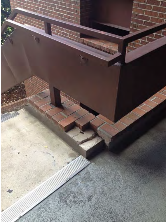
A15 – handrail base brick missing (several places)
