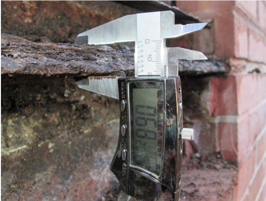
S21 - Caliper measurement of delaminated shelf angle leg (~0.68-inch)
