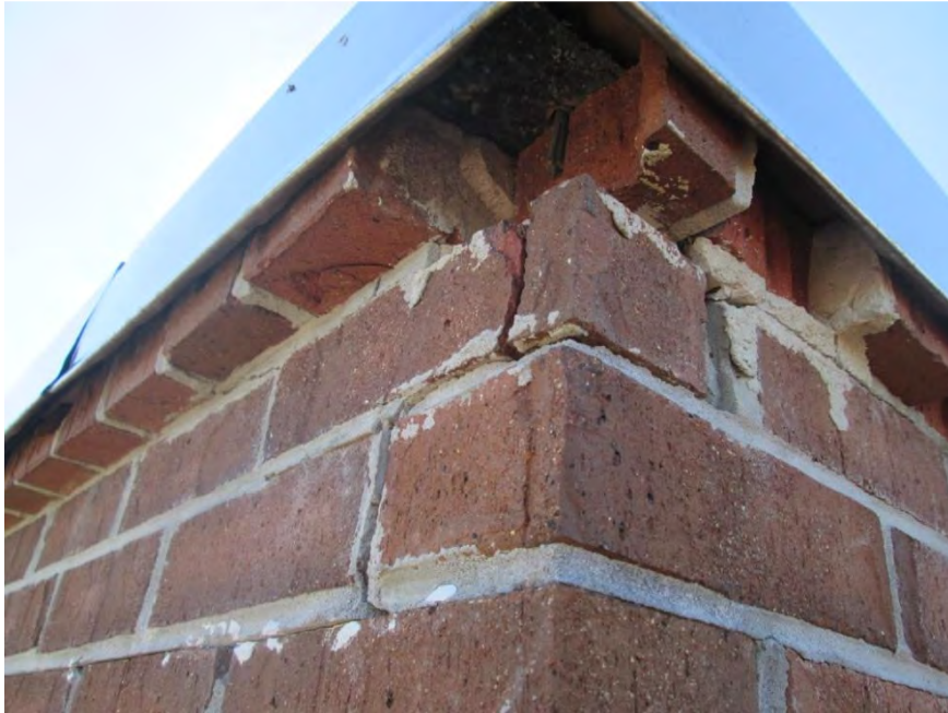
S3 - Cracked overhead brick noted beneath Roof Level parapet wall coping cap
