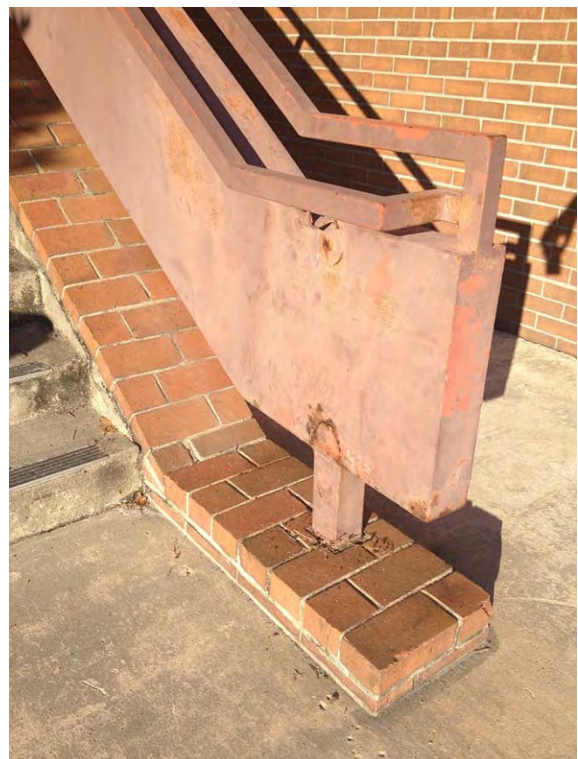
A14 – handrail corrosion
