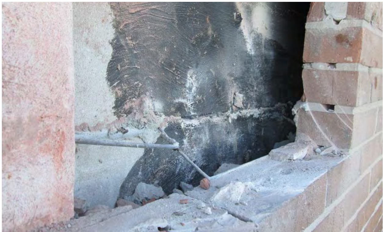
tower waterproofing – deteriorating and not consistently applied, brick ties not embedded in mortar
