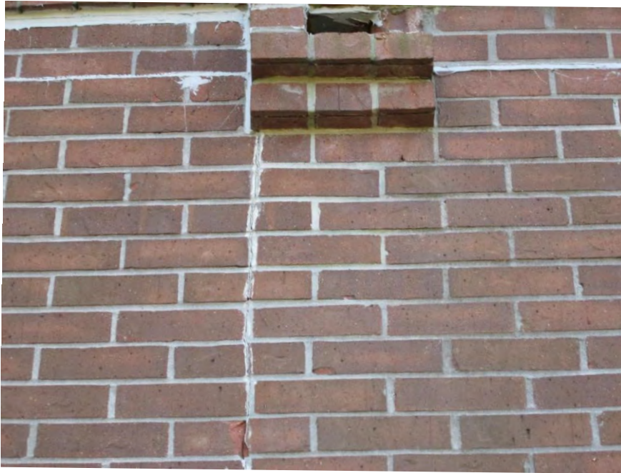
S11 - Cracked and spalled brick
