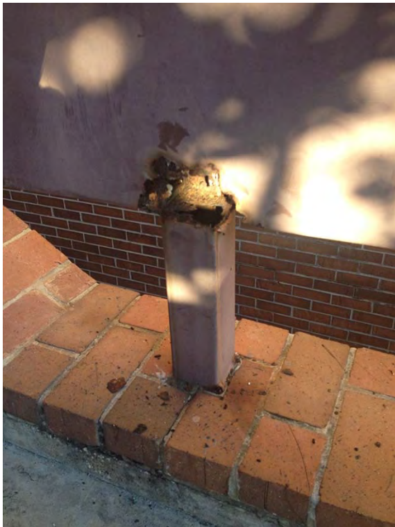
A13 – handrail corrosion
