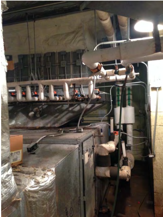
M1 – insufficient AHU coil pull clearance
