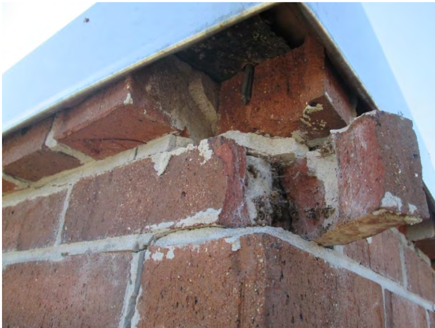
S4 - Cracked overhead brick shown in Photo S3 readily dislodged by hand
