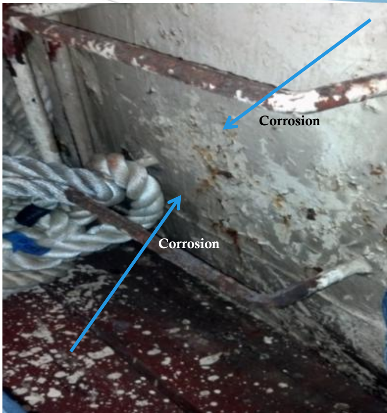
View: R/V Bellows Forepeak Bulkhead looking aft
